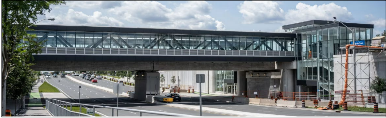
Figure 9: View of the Surrounding Premises - New rail overpass
