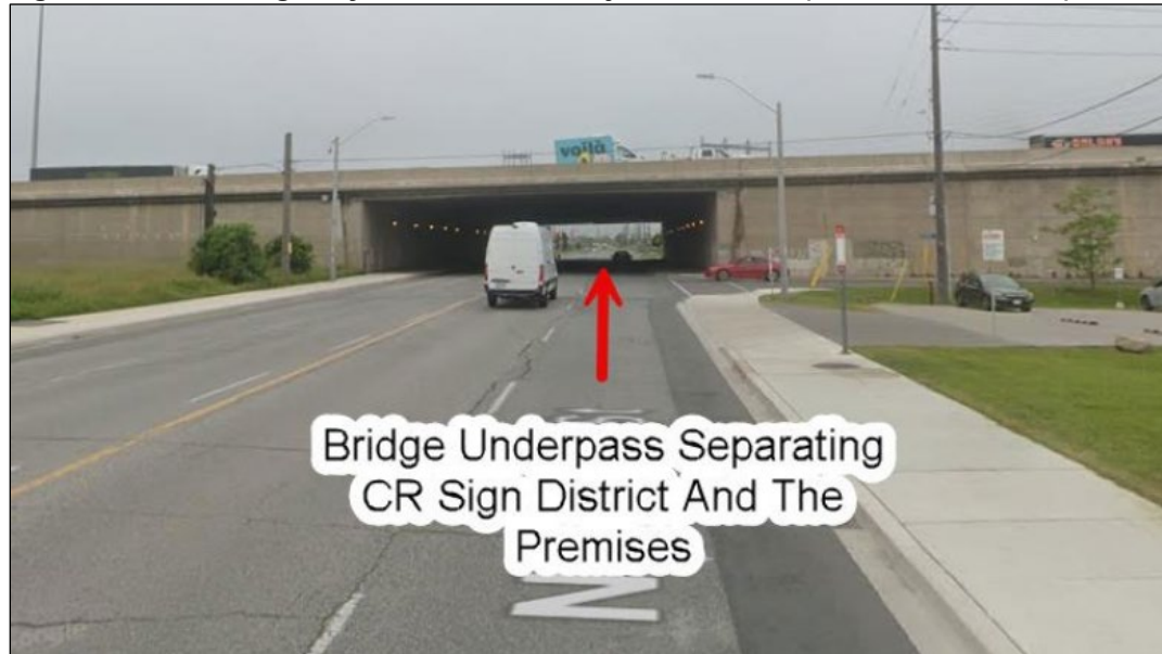
Figure 6: View of Highway 427 from the Subject Premises (from Submissions)
