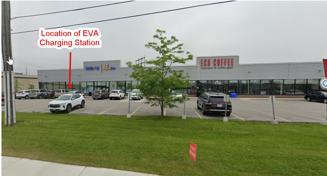
Image 1: Location of EVA Charging Station on the Premises
