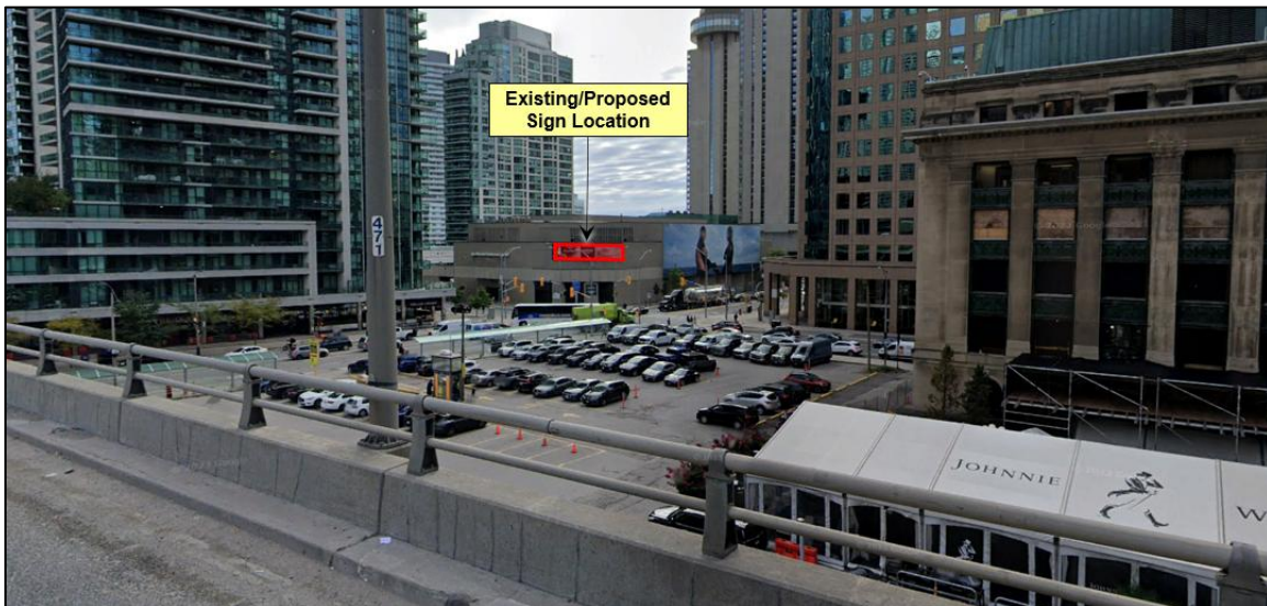
Figure 7: View from the F.G. Gardiner Expressway, facing southeast
