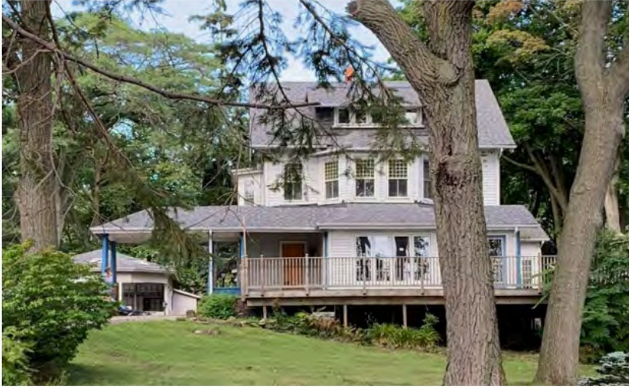
Figure 3: South elevation of 1 Fallingbrook Road, looking north (ERA Architects Inc.).
