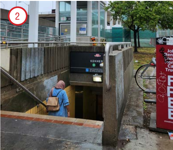
Figure 1.15 Existing Underground Connection
