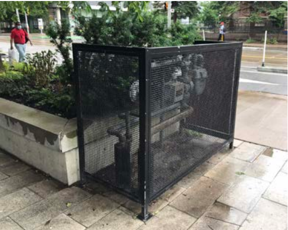
Figure 3.35 Decorative Screening for Utilities, Toronto, ON
