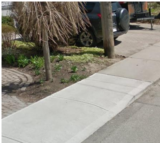
Permanent repairs completed – grinding or reconstruction
