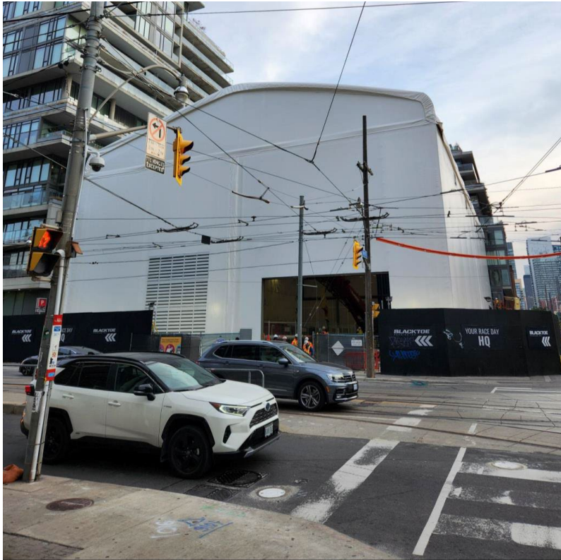
Figure 5: Exterior of King/Bathurst acoustic shelter (Source: Metrolinx)
