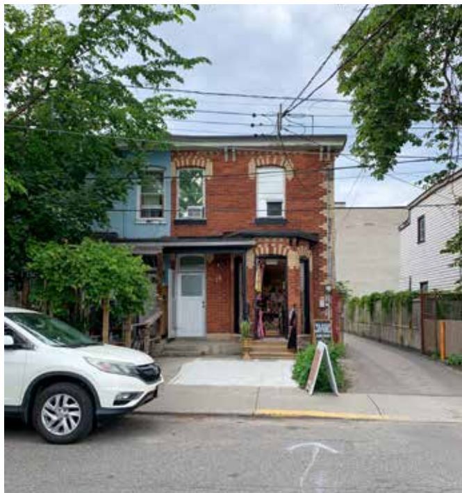
Figure 65: This conversion of a window opening into a door to accommodate commercial use of the ground floor at 78 Nassau Street conserves the legibility of the contributing property's architectural style and typology.
