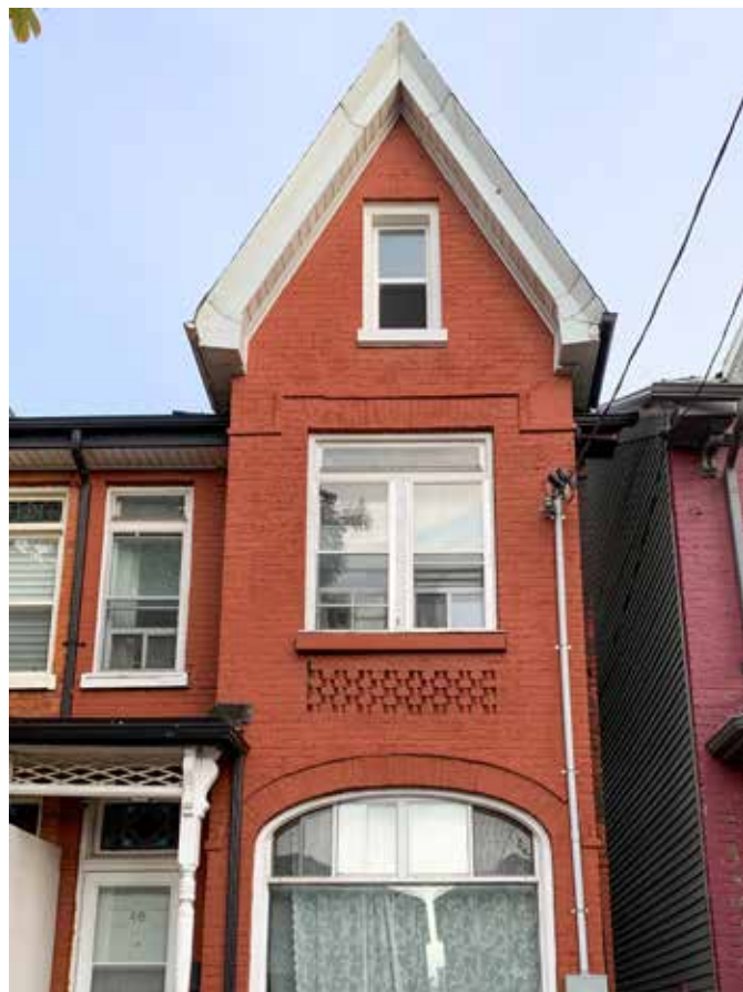
Figure 64: Example of patterned brickwork detail at 46 Nassau Street.
