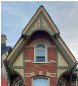
Figure 62: Wood trim detail on a Bay-and-Gable building on Kensington Avenue.
