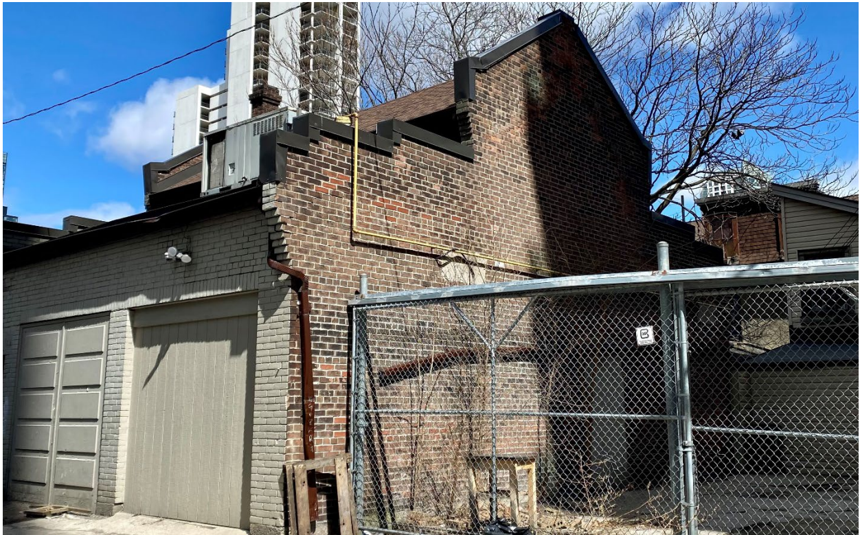
The rear coach house, viewed from Donna Shaw Lane, 2022 (Heritage Planning).
