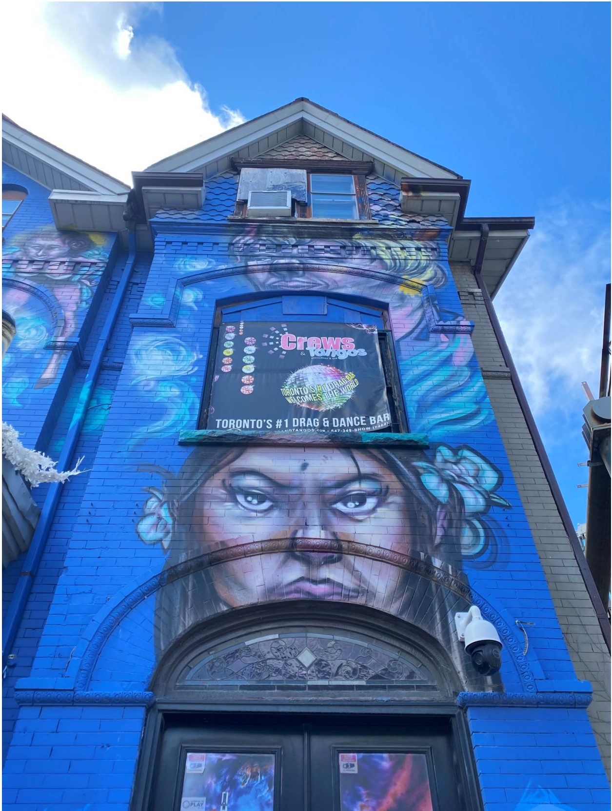
Architectural detailing on the northernmost bay of the front elevation, 2022 (Heritage Planning).
