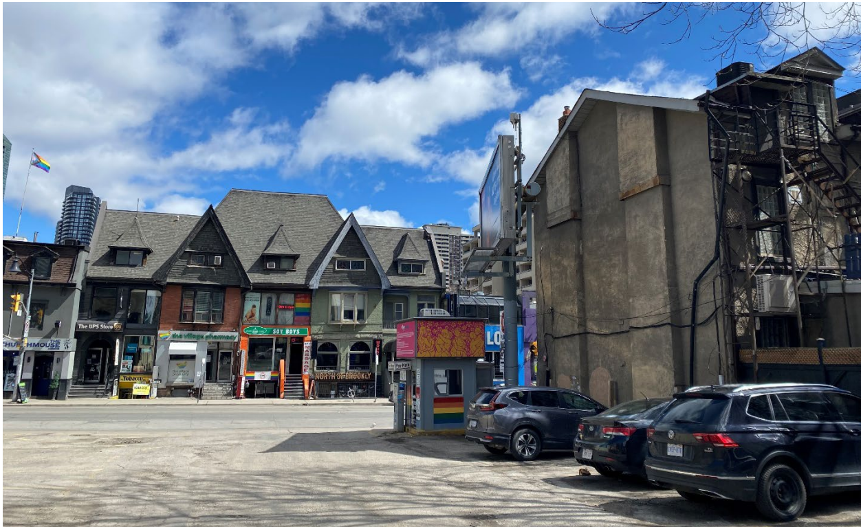
Eastward view from the parking lot immediately north of the subject properties, with the north and rear building elevations visible at right, 2022 (Heritage Planning).
