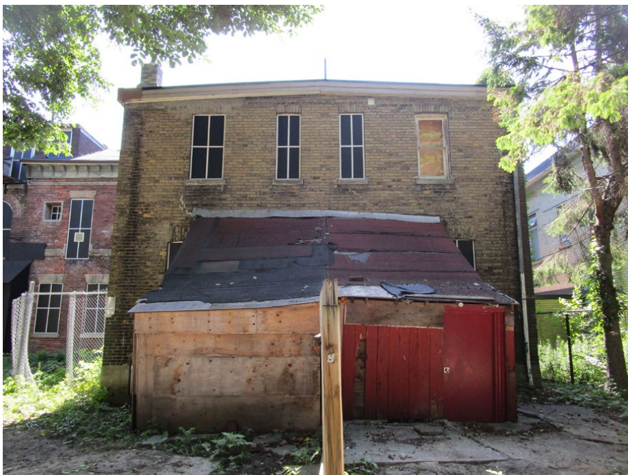
309-311 George St - east elevation (ERA)
