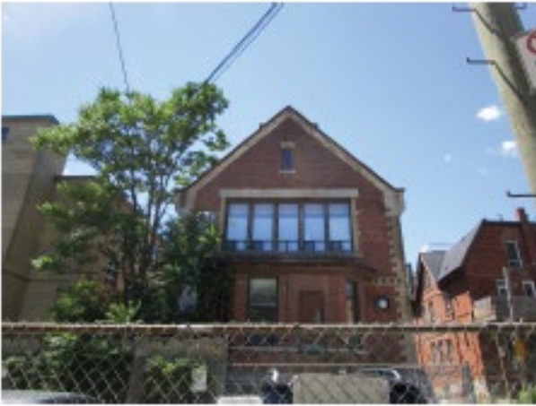
East elevation of 349 George Street (ERA)
