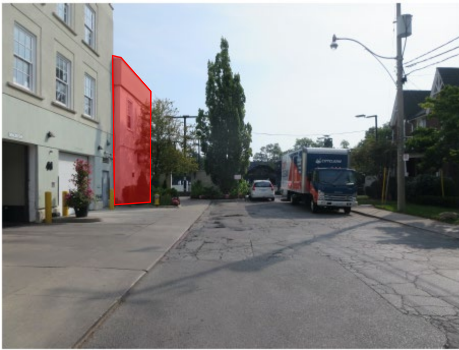
Photograph of Price Street showing the south elevation of the portion of 44 to be demolished (highlighted in red). (Source: GBCH)
