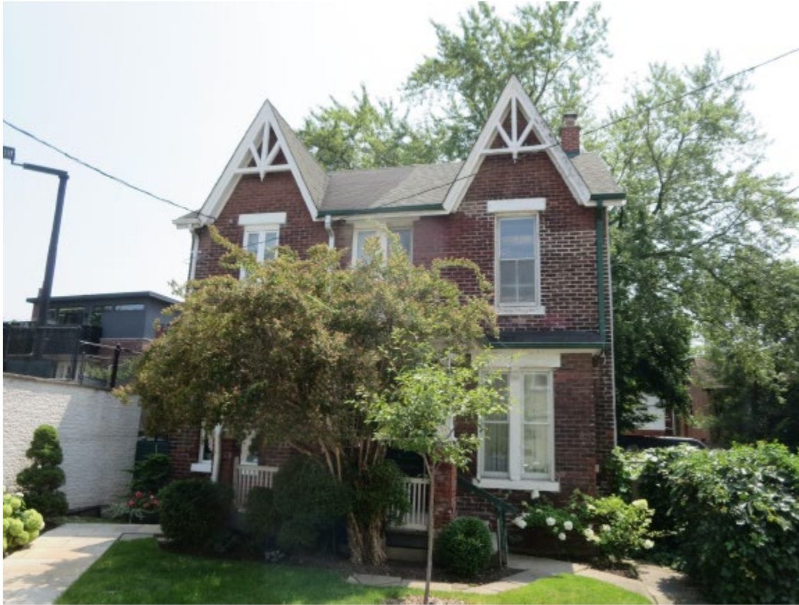
Photograph of the north elevation (front) of 43-45 Price Street. (Source - GBCH)
