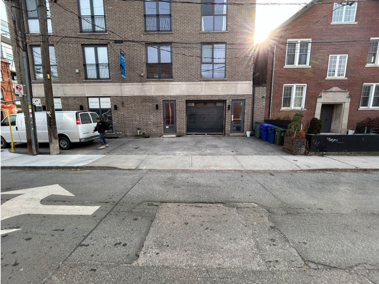
Attachment 3: Proposed encroachment location within the boulevard, view from Argyle Street - 114 Ossington Avenue
