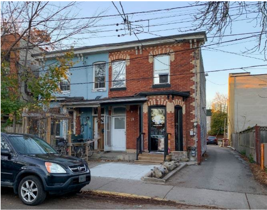
78 and 80 Nassau Street (Heritage Planning, November 2024).
