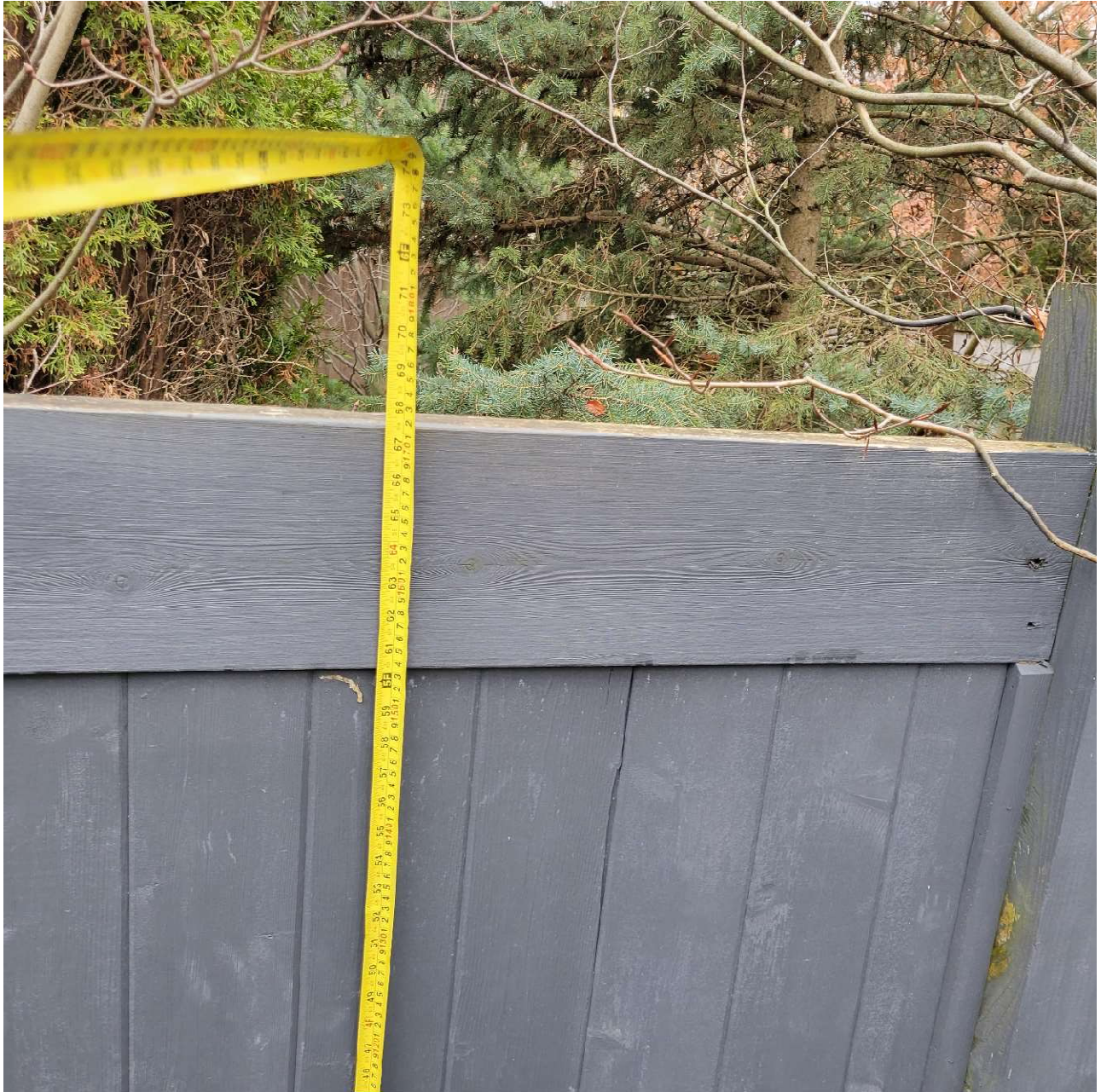
Attachment 9: Photograph depicting wooden perimeter pool enclosure fence on the east side of property, measured at 1.72m.
