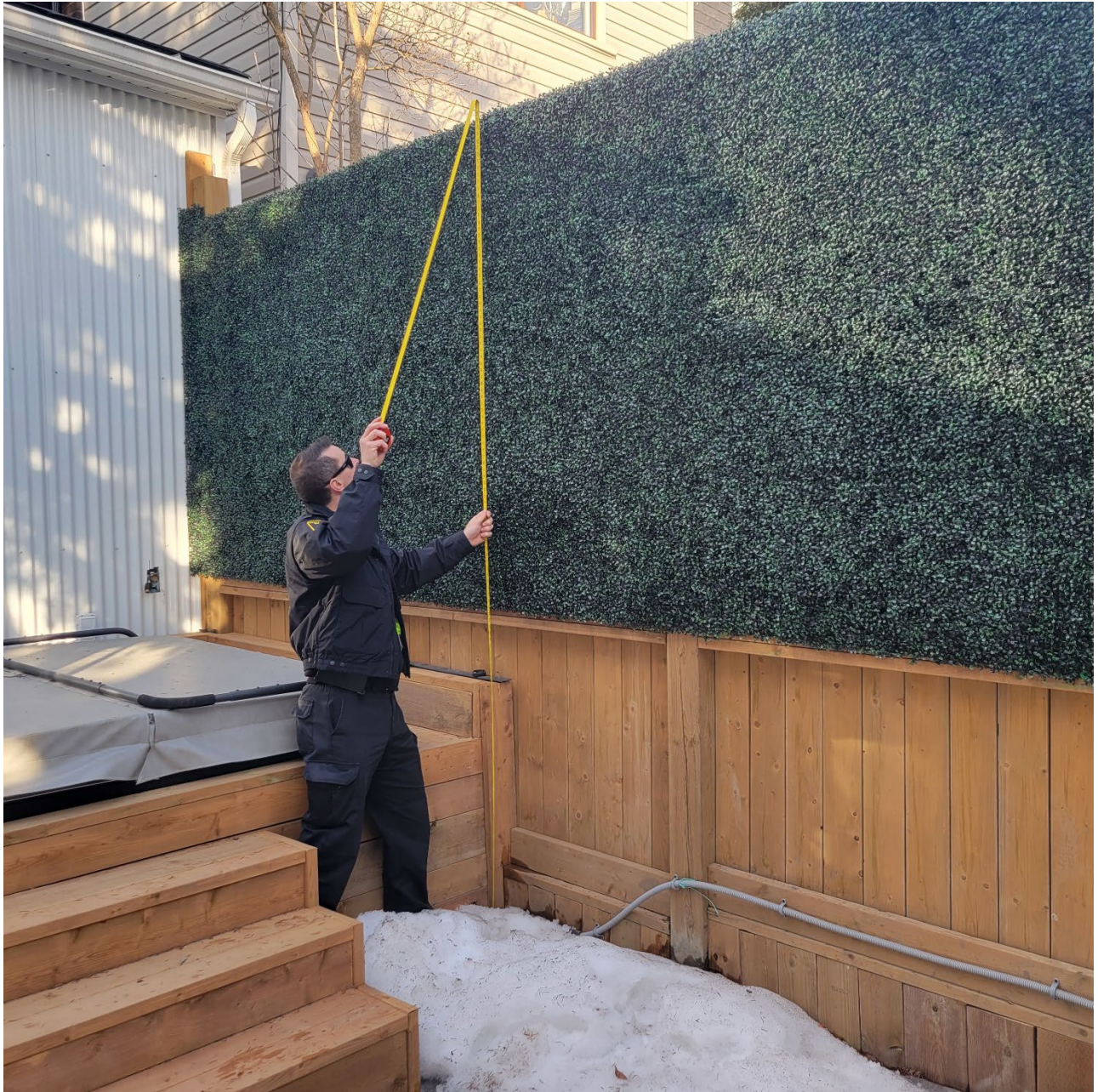
Attachment 9: Photograph depicting existing northern fence, of 3.14 metres in height. Maximum height for the fence is 2m.
