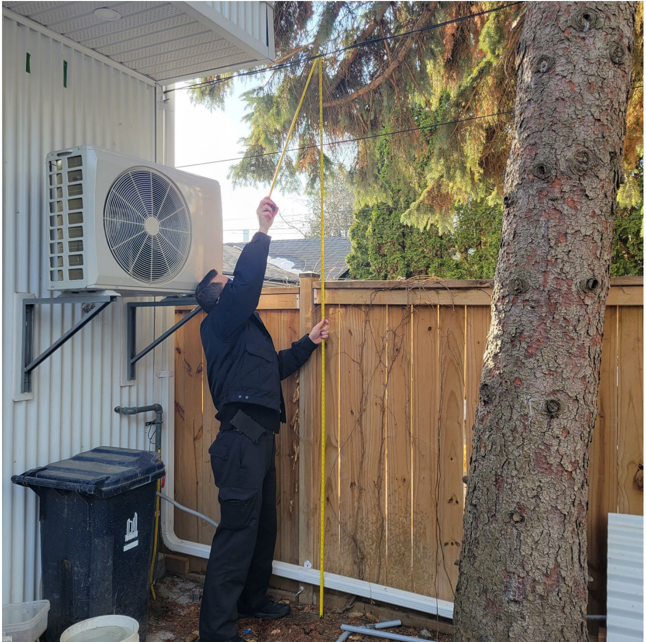
Attachment 14: Photograph depicting proposed southern fence, of 3.10 metres in height. Maximum height for the fence is 2m.
