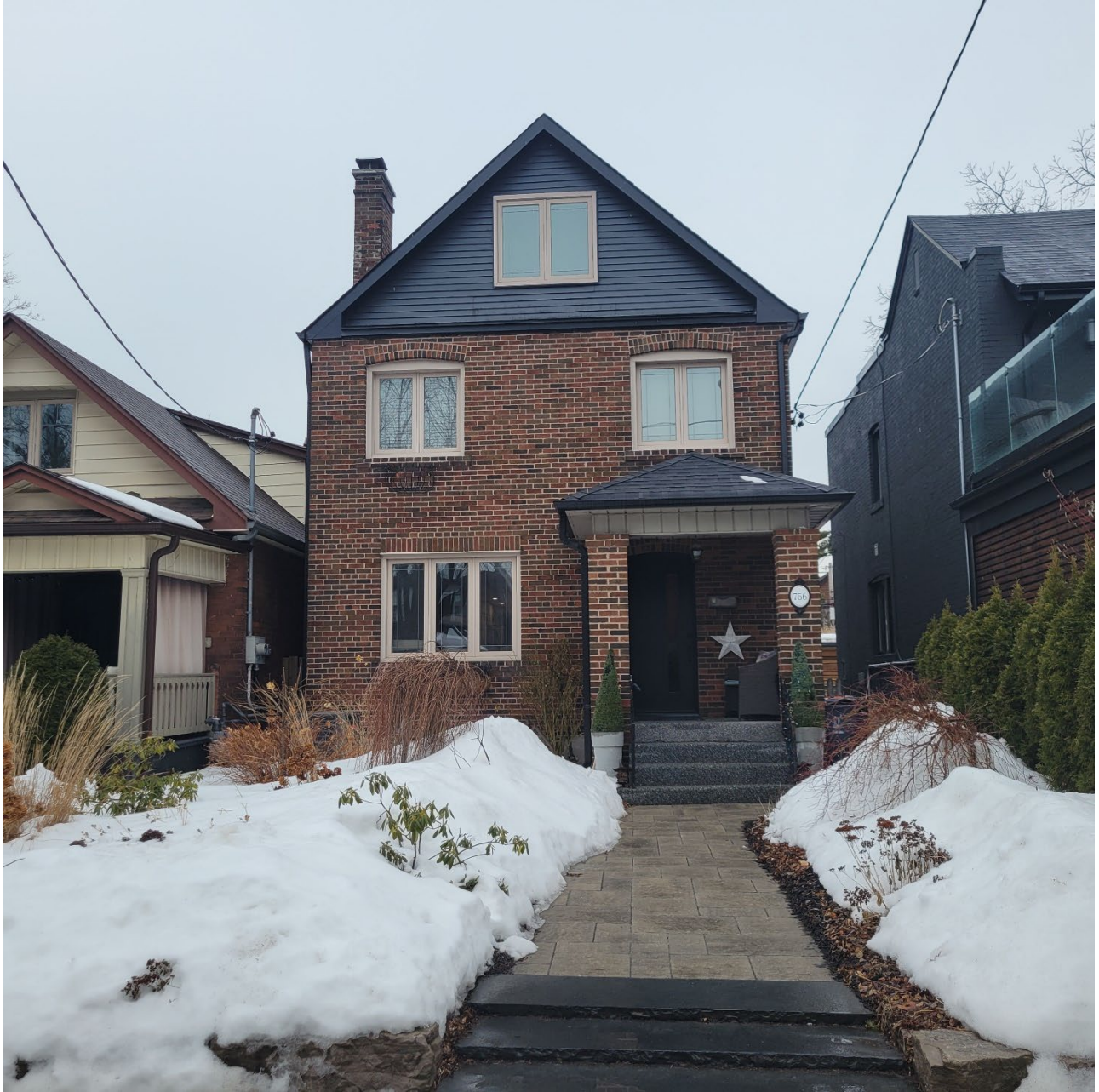
Attachment 4: Photograph of the front of property, 756 Windermere Ave. Photograph taken from Windermere Ave.
