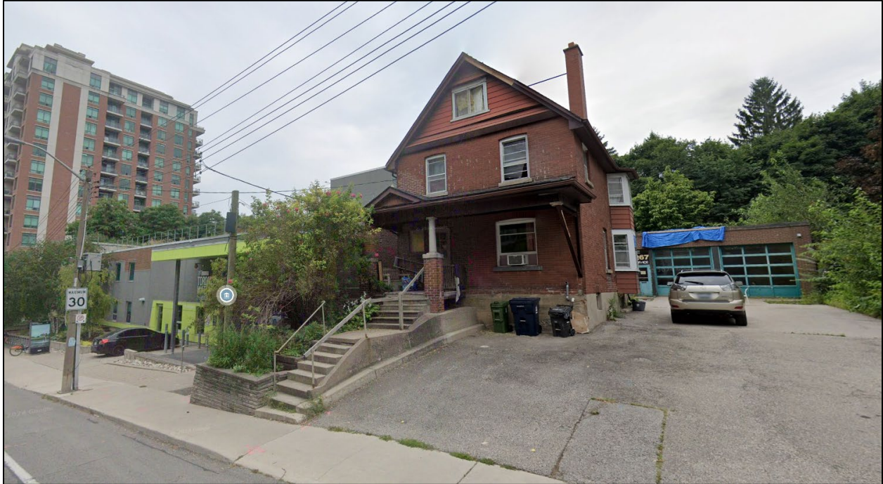
Photo 1: 267 and 275 Merton Street
