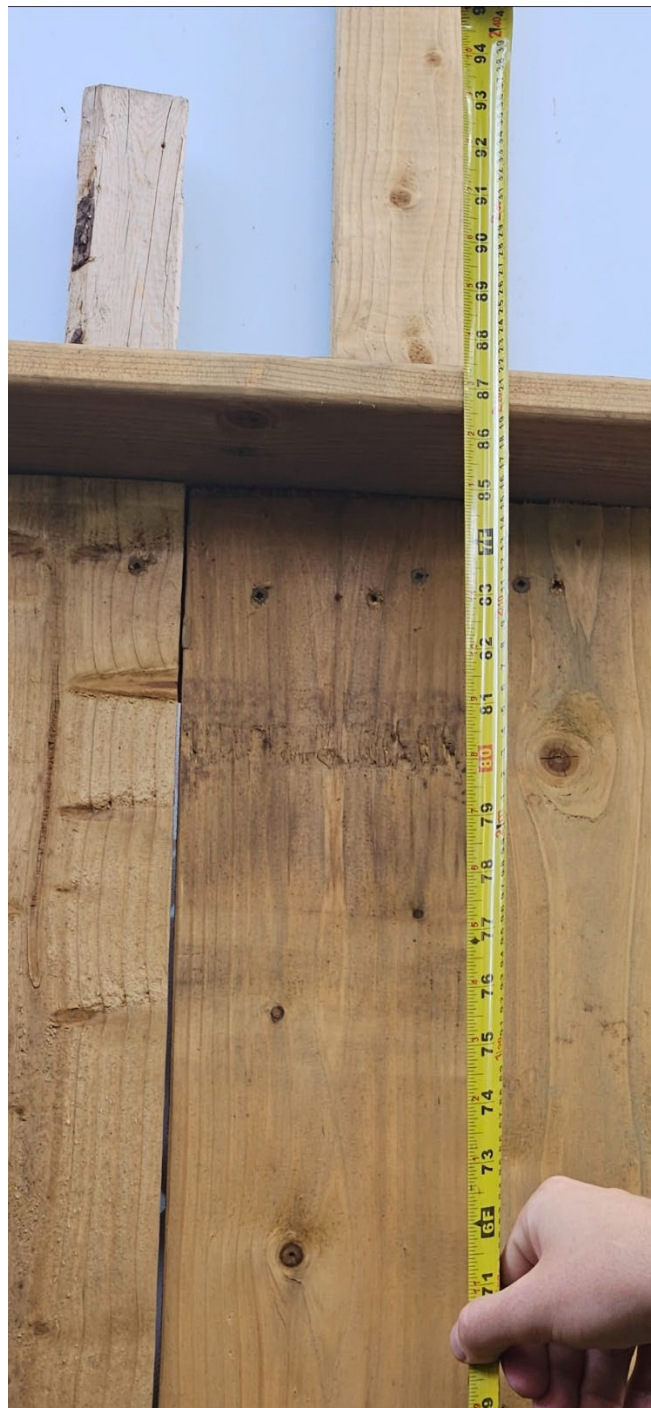
Attachment 10: Officers photo [Measurement taken from grade to top of the west section of fence 2.22m]
