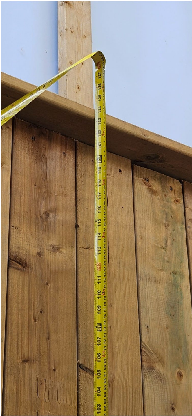
Attachment 7: Officers photo [Measurement taken from grade to top of the east section of fence 3.15m]
