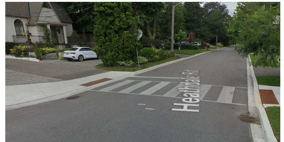
Heathdale Road and Raglan Avenue, where a portion of the driveway provides the sidewalk ramp.
