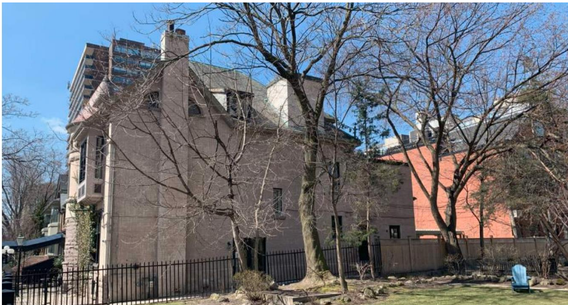
East elevation of 36 Prince Arthur Avenue showing existing windows, chimney, elevator overrun to be altered (Source: ERA Architects Inc., 2024)
