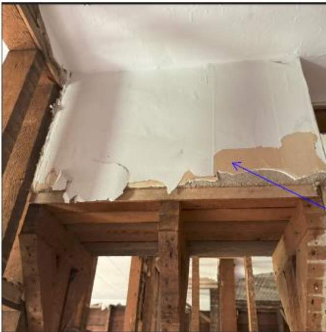
Joist floor Damage
