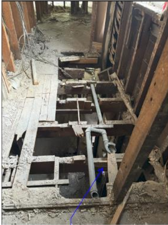
Joist floor Damage
