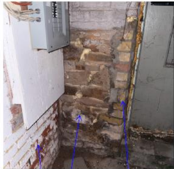
Multiple material in foundation walls
