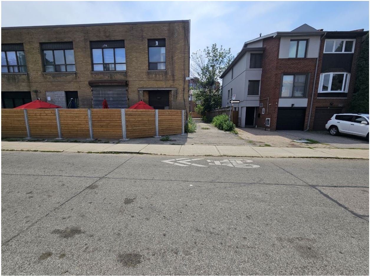
Flank of 629 Adelaide St W, looking south at the north-south lane
