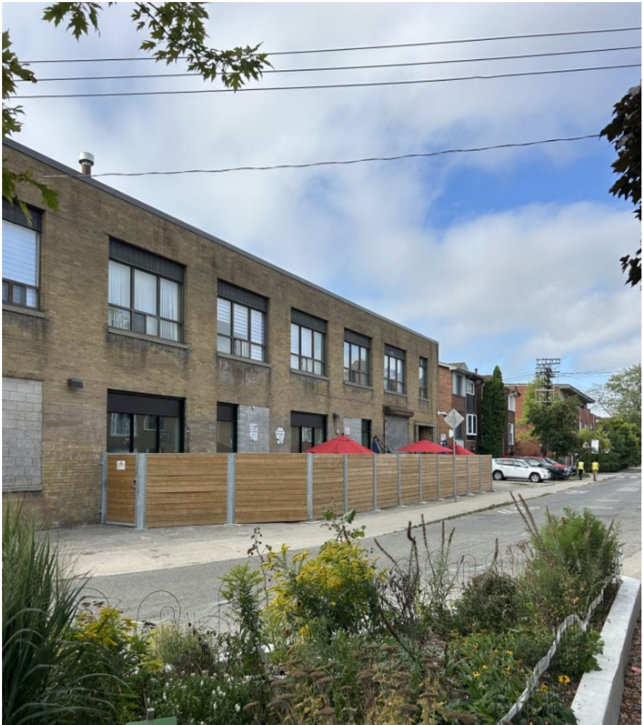
Flank of 629 Adelaide St W, looking southwest
