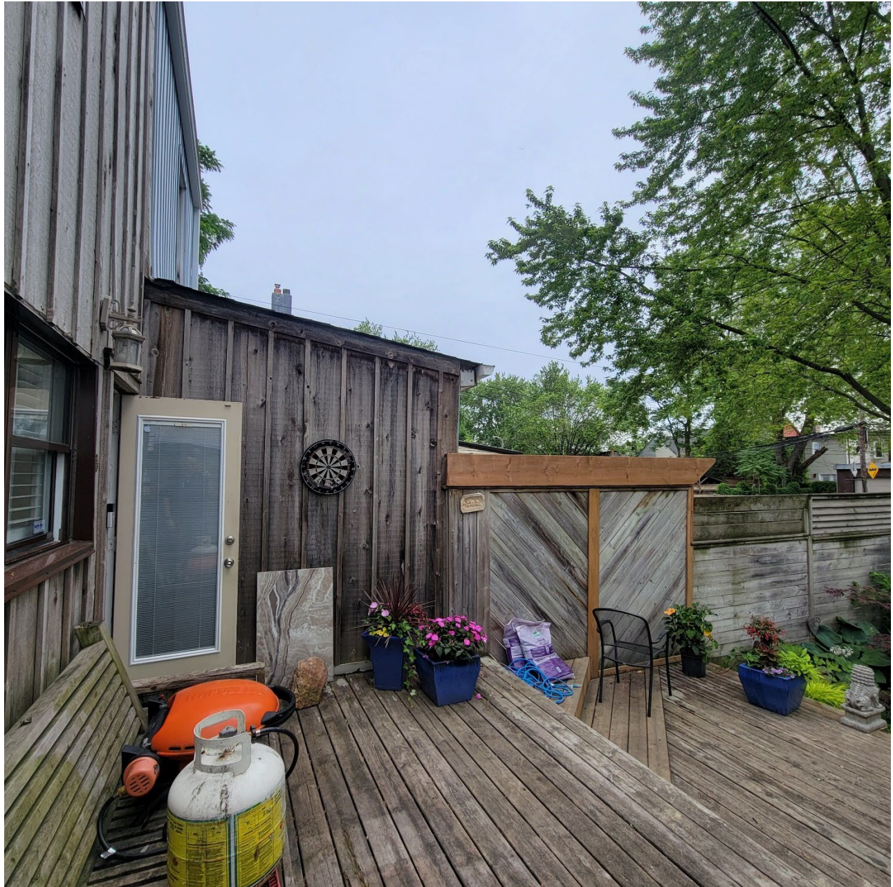
Attachment 7: Photograph depicting existing north property line fence.
