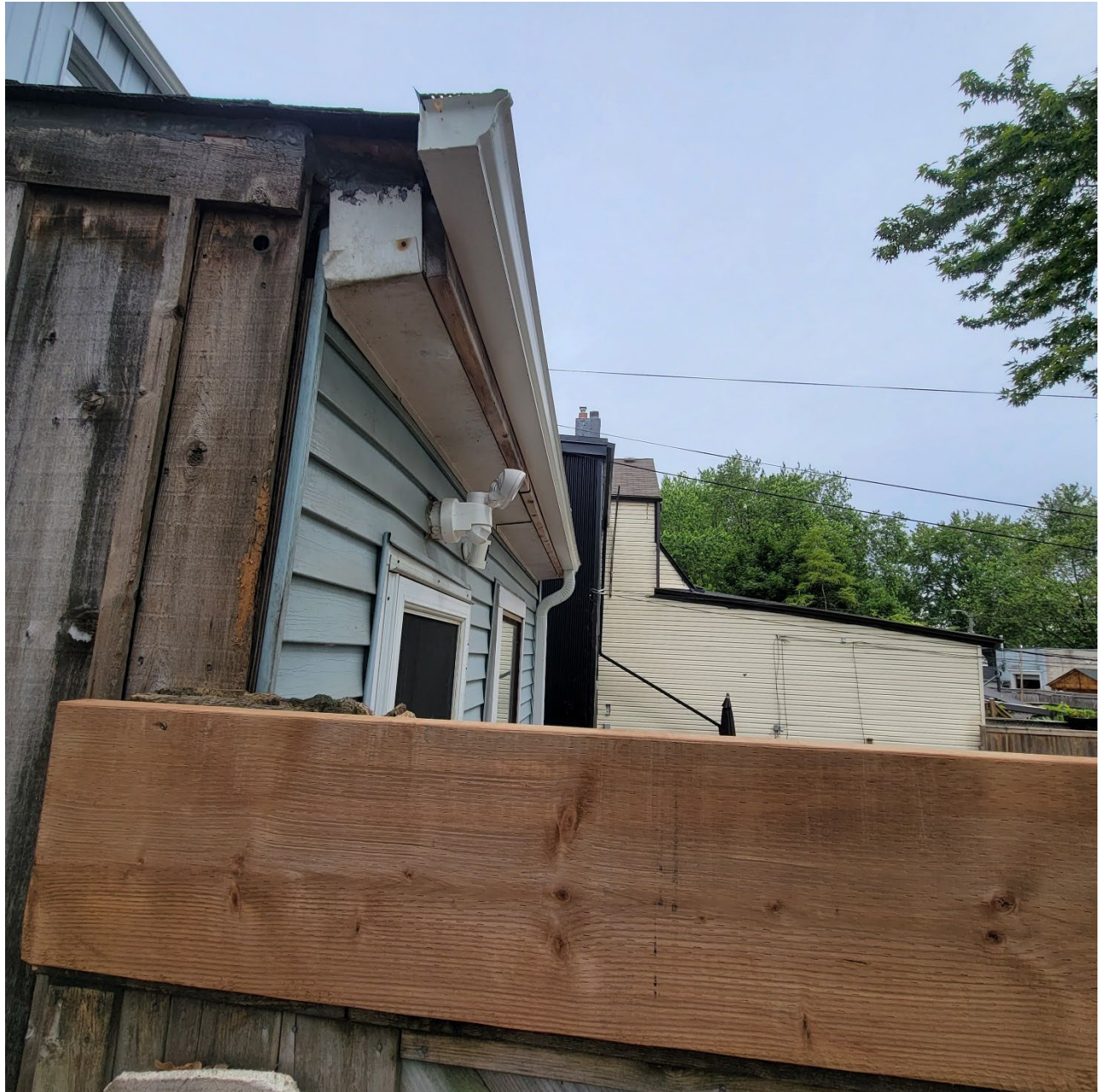
Attachment 8: Photograph depicting existing north property line fence.
