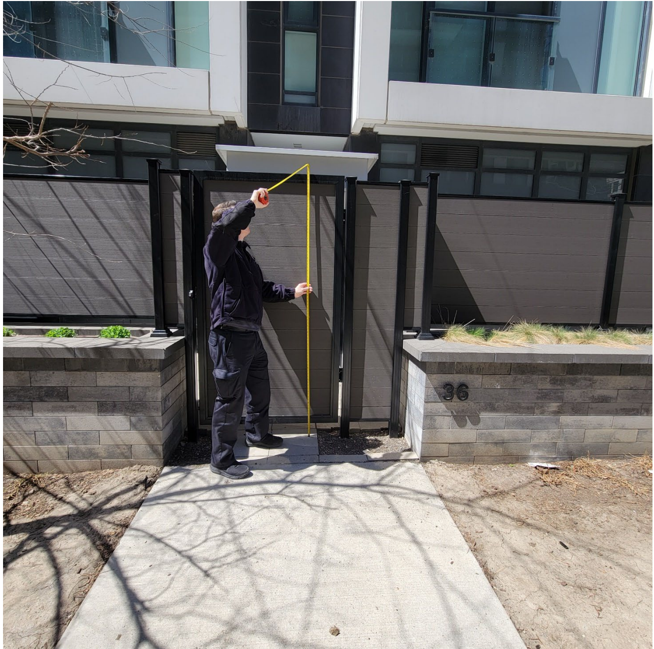
Attachment 20: Photograph depicting measurement of 2.17 meters from grade to the top of the gate at 36 Tubman Ave. Maximum height is 1.2 meters .
