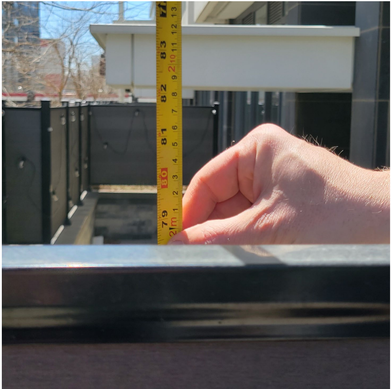
Attachment 28: Photograph depicting height measurement of 2.0 meters from grade to the top of the fence. Maximum height is 1.2 meters .
