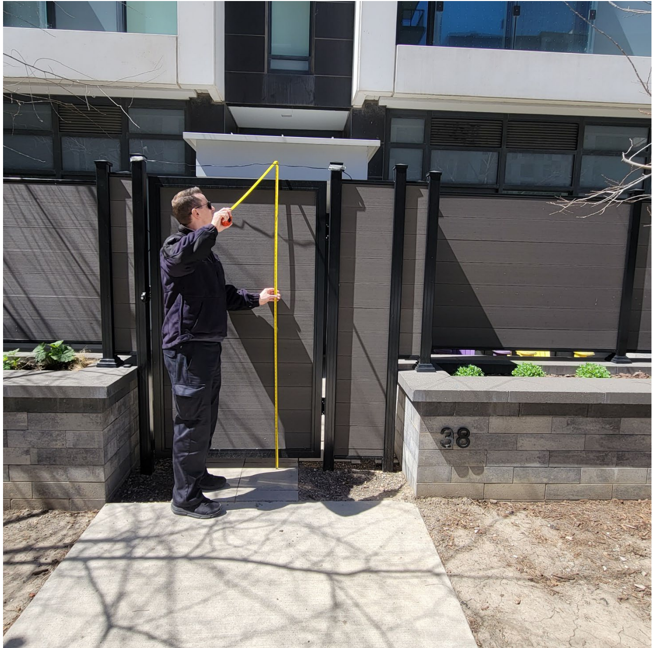
Attachment 22: Photograph depicting measurement of 2.02 meters from grade to the top of the gate at 38 Tubman Ave. Maximum height is 1.2 meters .
