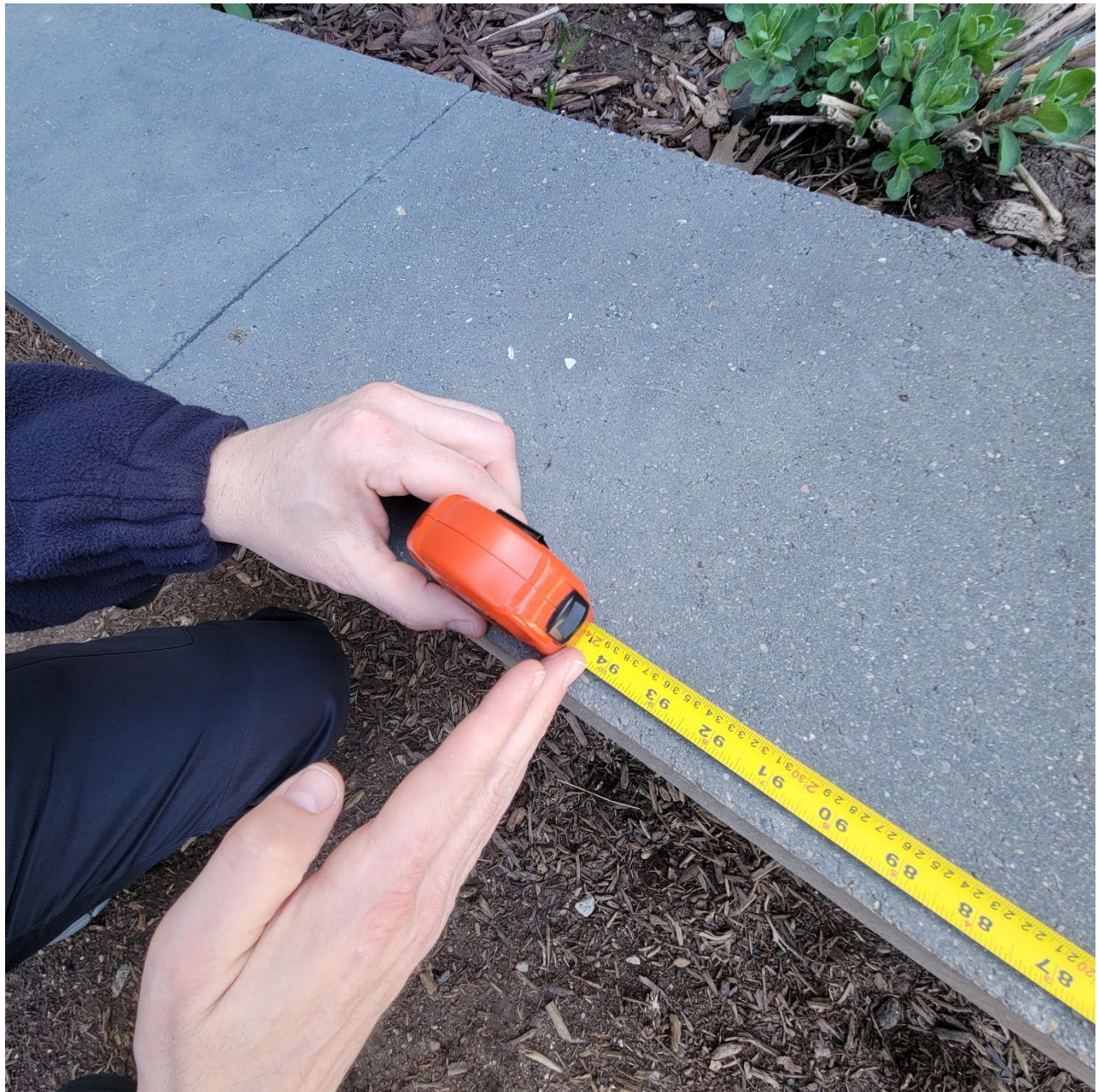
Attachment 13: Photograph depicting measurement of 2.4 meters from front lot line. Maximum height is 1.2 meters within this measurement.
