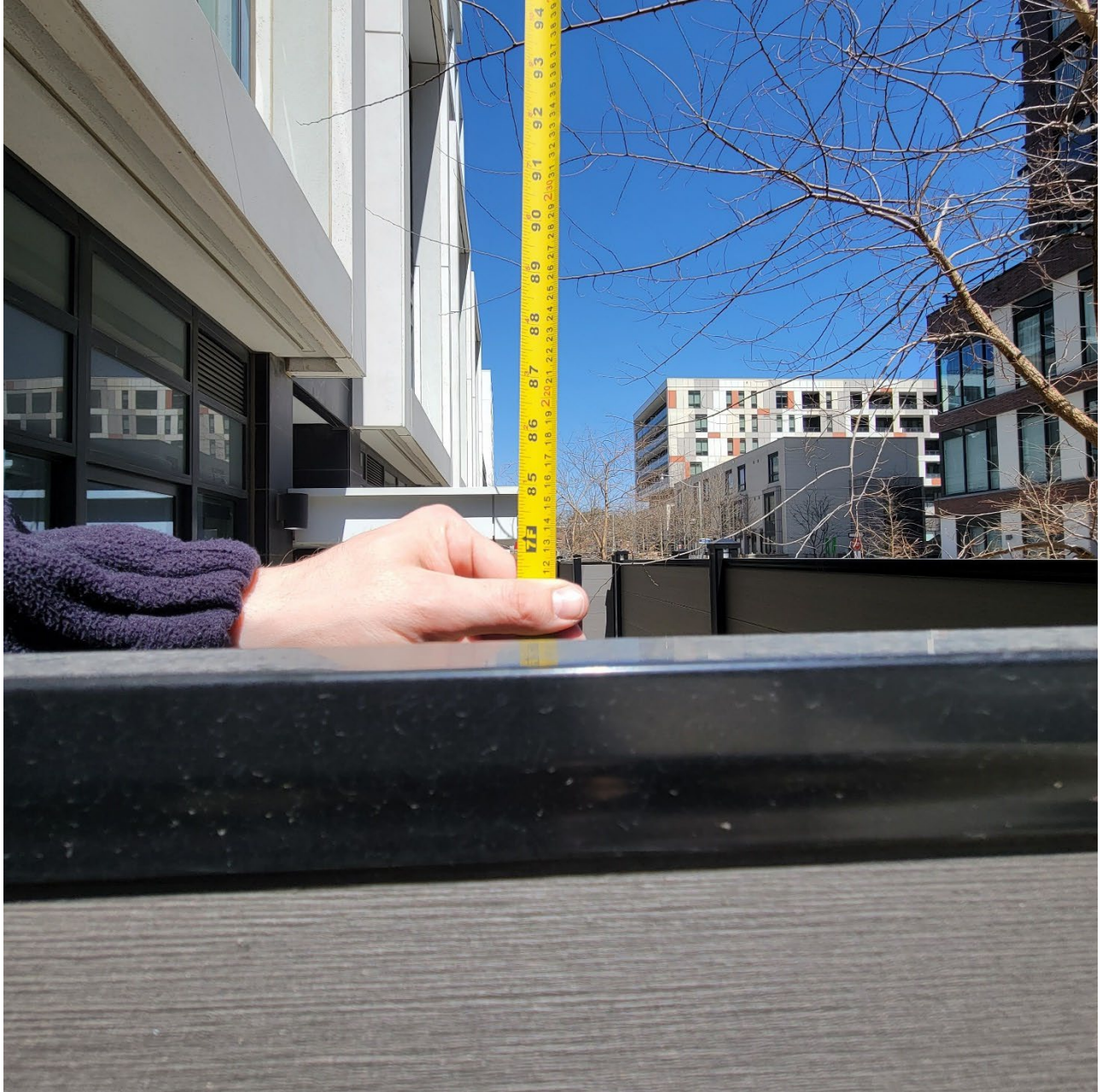
Attachment 19: Photograph depicting height measurement of 2.12 meters from grade to the top of the fence. Maximum height is 1.2 meters .
