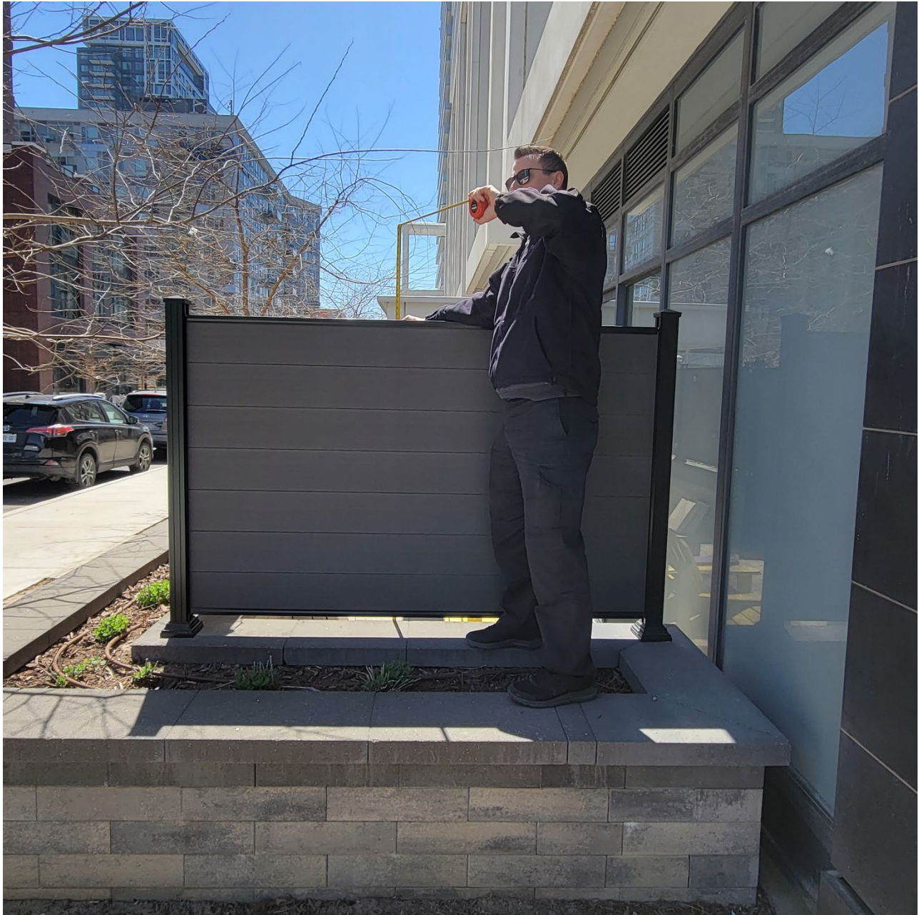
Attachment 27: Photograph depicting height measurement of 2.0 meters from grade to the top of the fence. Maximum height is 1.2 meters .
