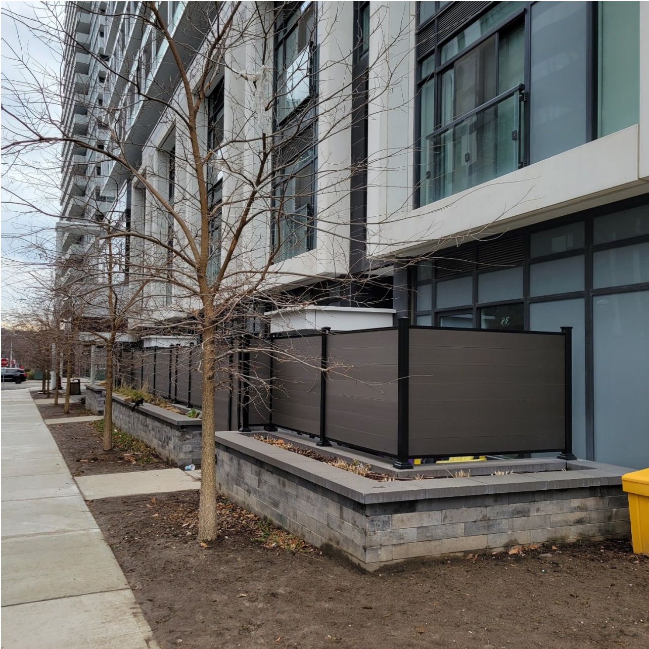
Attachment 24: Fence on the east side of the property, flanking Tubman Ave, looking south, lower masonry and upper aluminum/composite fence
