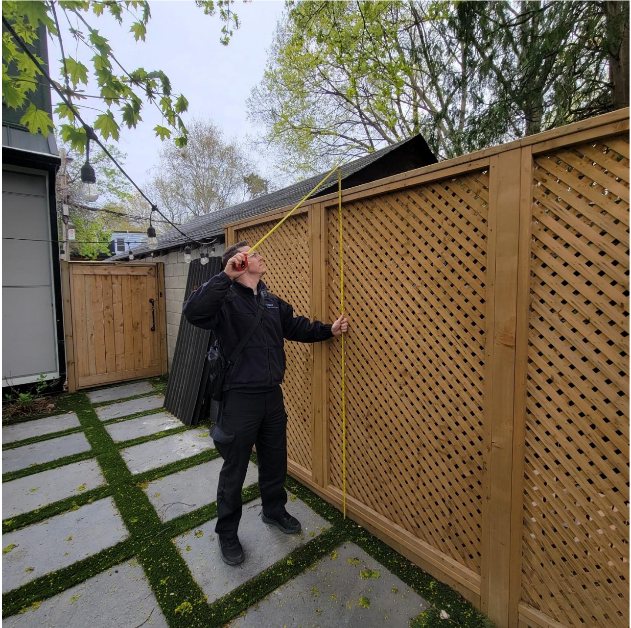
Attachment 12: Photograph depicting the measurement of the south side perimeter fence of the rear yard of 47 Lewis St., (2.26 metres through rear yard adjacent to the laneway suite)
