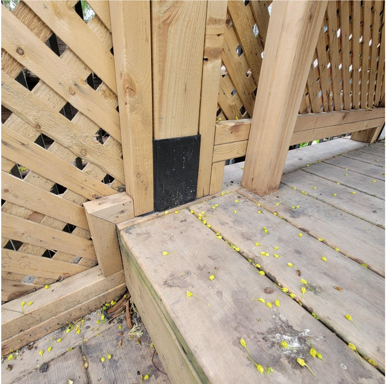
Attachment 14: Photograph depicting the on-deck, fence post base-bracket of the south side perimeter fence on the rear yard of 47 Lewis St., (2.48 metres surrounding the rear deck)
