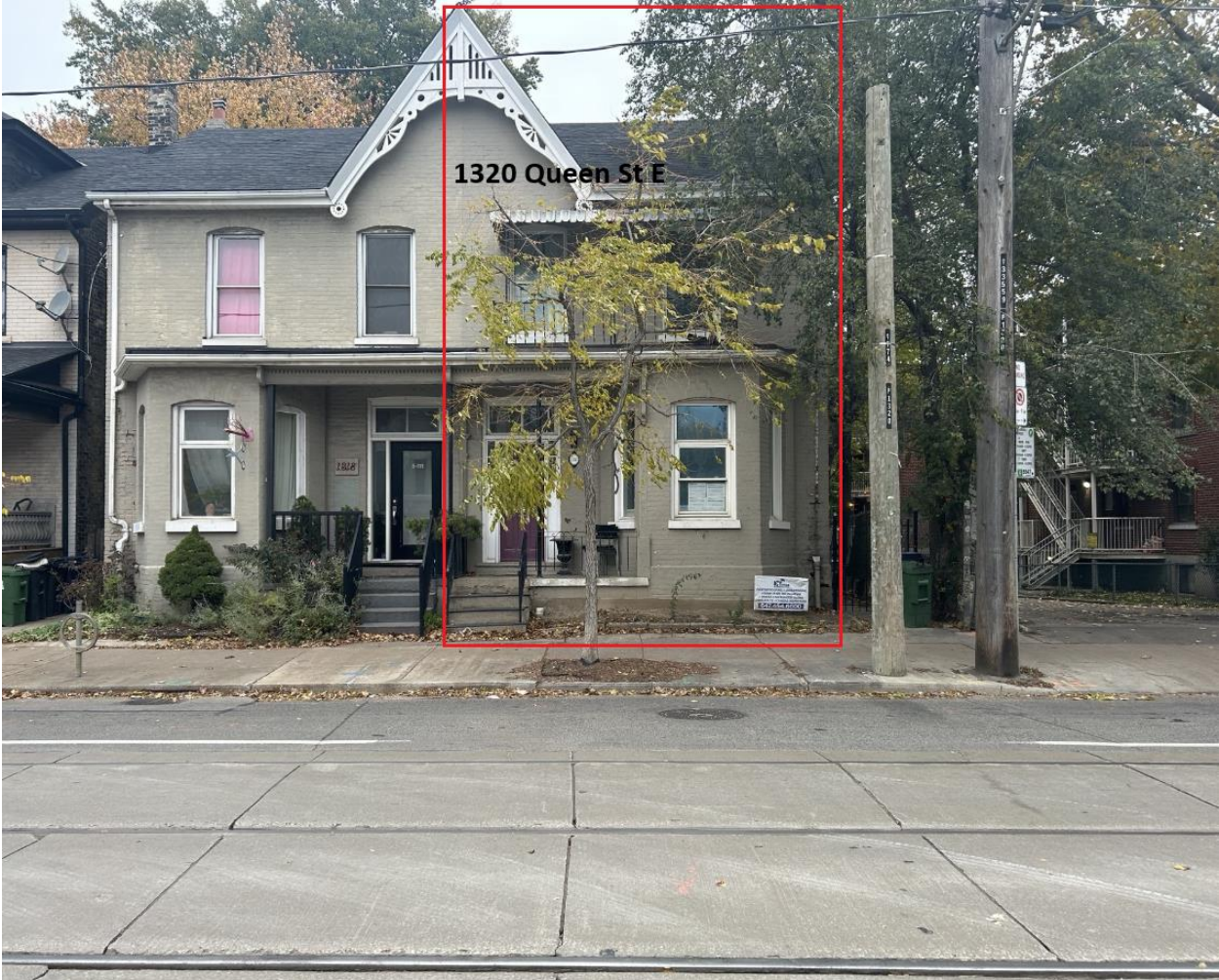
Looking north at 1320 Queen Street East
