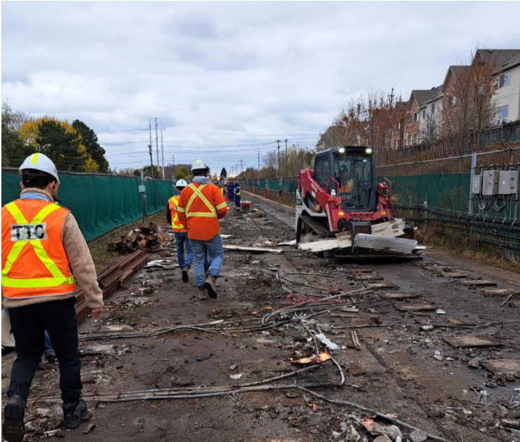
Above: Track removal on Line 3.
