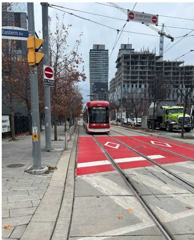
Figure 4: Red-paint application at dedicated streetcar right-of-way entrance (at Cherry/Eastern)
