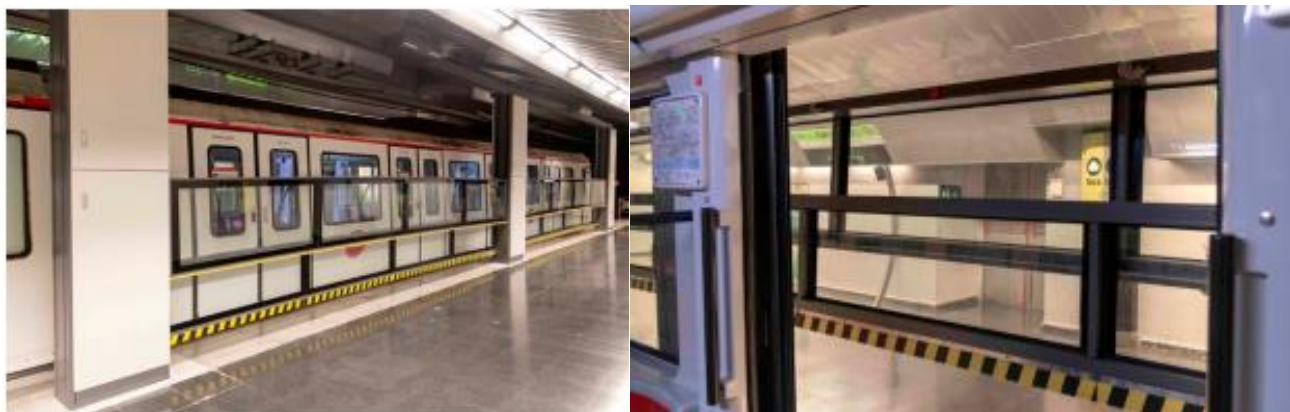
Figure 44: Vertical PED trials at Barcelona Metro [14]
