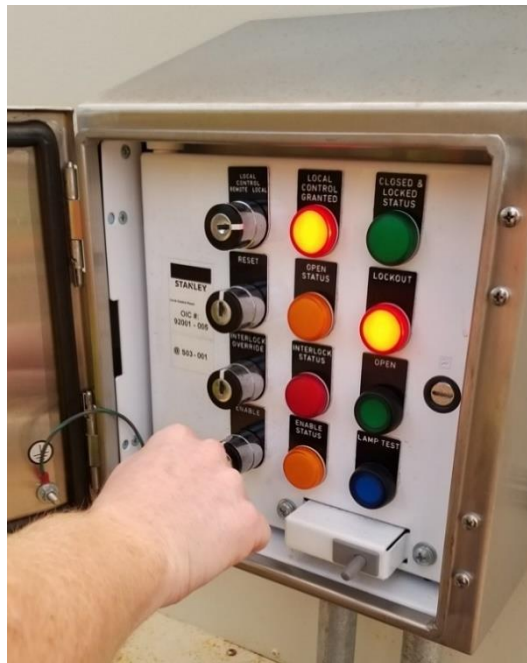
Figure 12: Example of a Local Control Panel from Stanley
