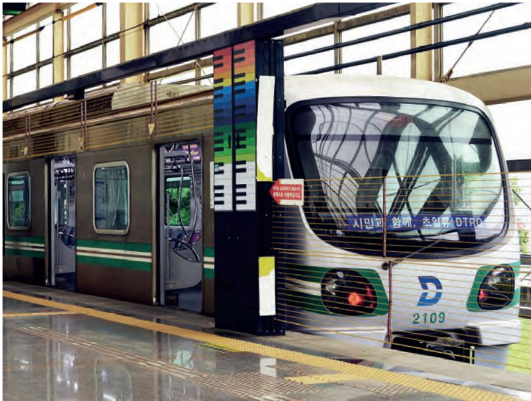
Figure 20: Rope Screen Door installation at Munyang Station in South Korea
