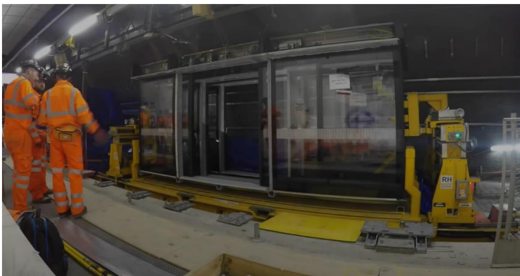
Figure 15: Workers using a customized work car to lift preassembled PED sections into place
