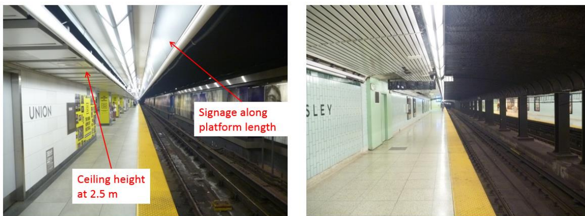
Figure 39: Lower platform ceiling height and increased obstruction by signage at Union (left) compared with Wellesley (right)
