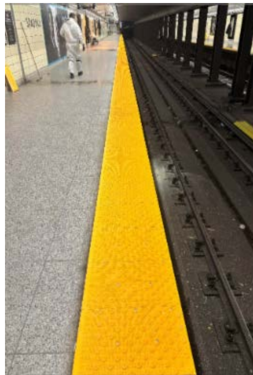
Above: Platform Edge Marker (PEM) work at Spadina Station.
