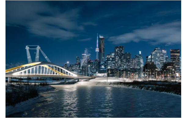
Continued Investment in Infrastructure
