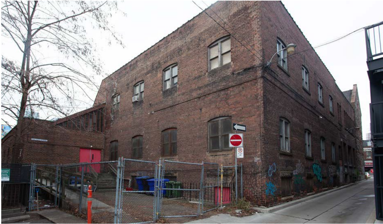
View of the east and south elevations of the 1912 Sunday school addition at 353 Sherbourne, looking north-west from laneway (ERA Architects)
