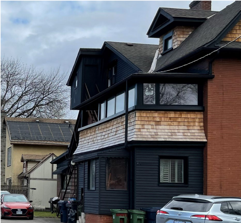
Figure 4: North (rear) elevation - oblique view from the northwest, 2025 (City of Toronto Heritage Planning)
