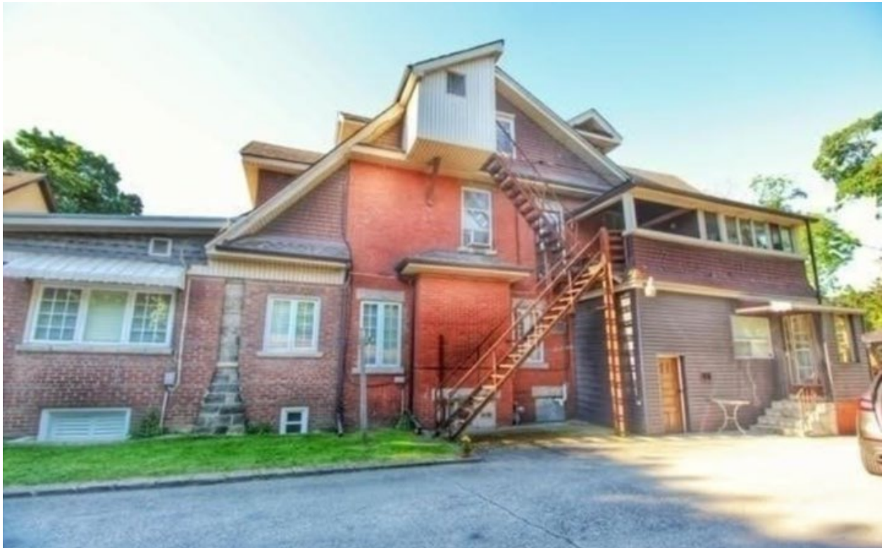
Figure 6: North (rear) elevation - historic verandah supports within the 1955 alterations (Royal Lepage Signature Realty, Brokerage 2021)
