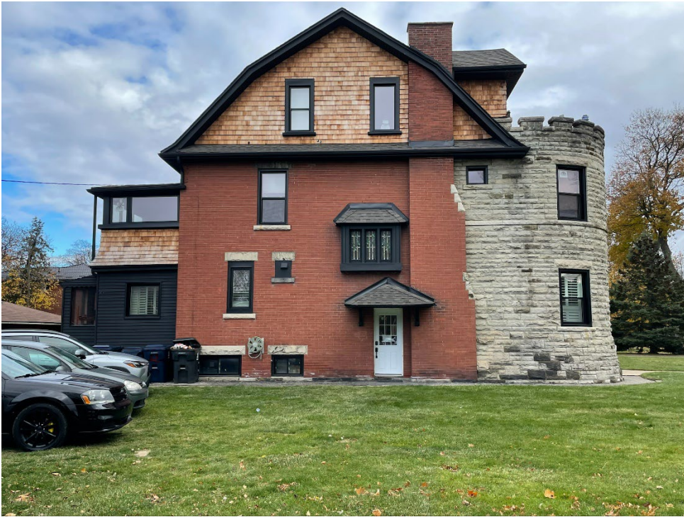
Figure 3: West elevation, 2025 (City of Toronto Heritage Planning)
