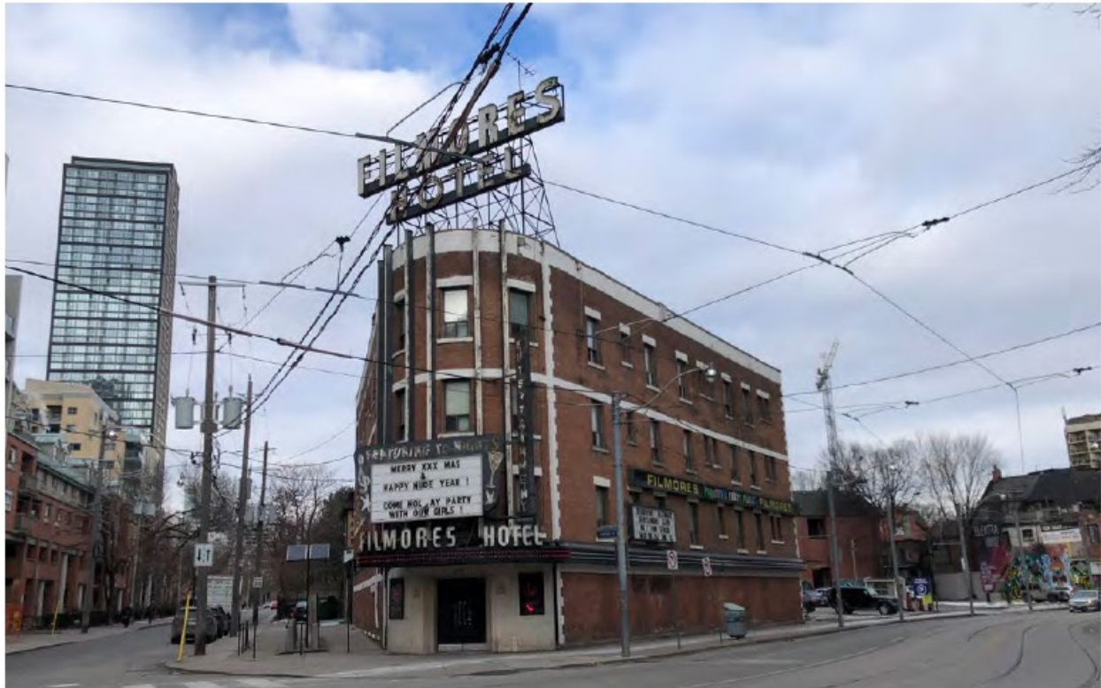
Figure 3: Photo of the south elevation of the existing building at 212 Dundas Street East (Giaino + Associates Architects Inc., 2025).
