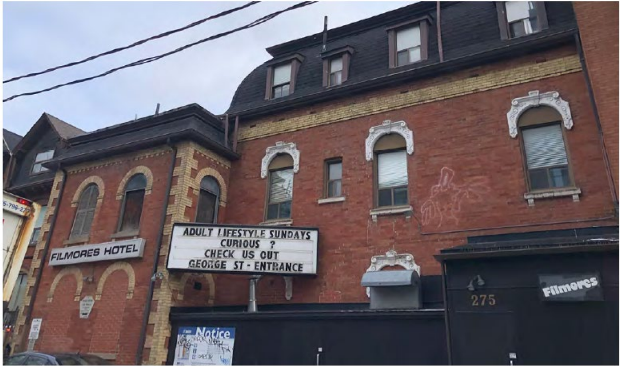
Figure 6: Photo of the west elevation of the existing building at 275 George Street (Gaimo + Associates Architects Inc., 2025).
