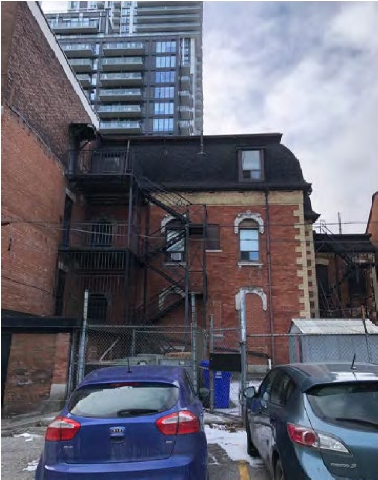
Figure 7: Photo of the east elevation of the existing building at 275 George Street (Giaino + Associates Architects Inc., 2025).
