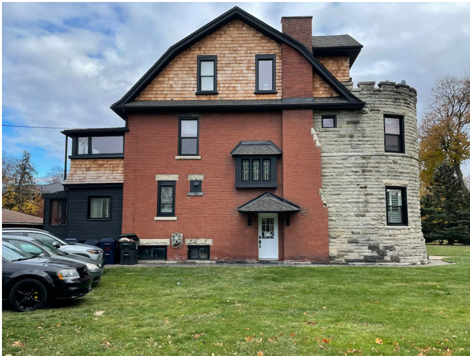
Figure 3: West elevation, 2025 (City of Toronto Heritage Planning)
