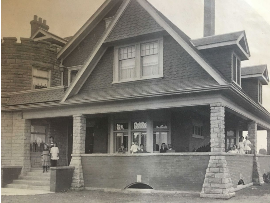
Figure 1: Historic view from the southeast showing the original wraparound verandah configuration and patterned shingle gable cladding, 1912 (Weston Historical Society)
