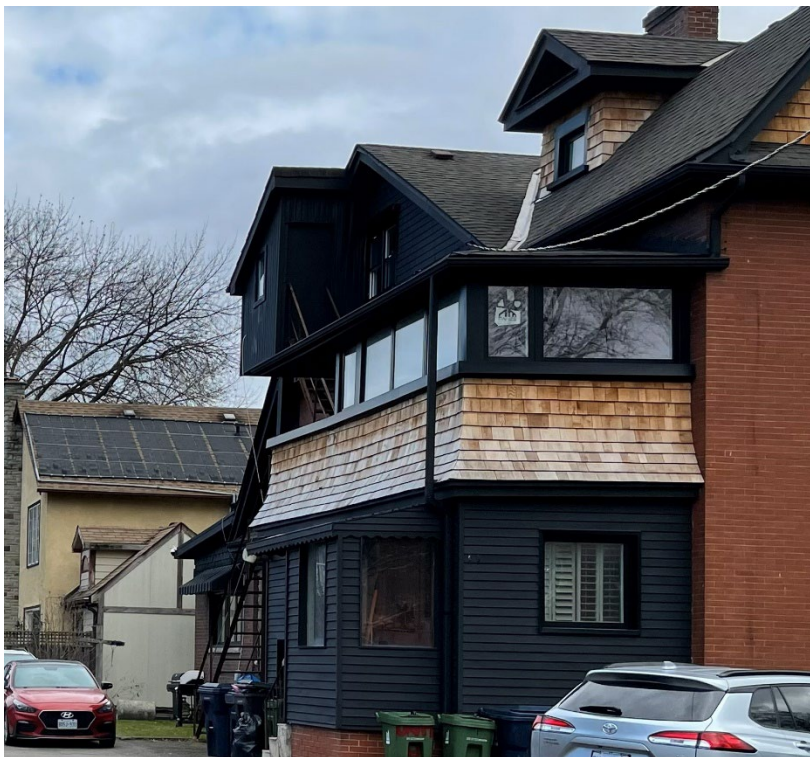
Figure 4: North (rear) elevation - oblique view from the northwest, 2025 (City of Toronto Heritage Planning)
