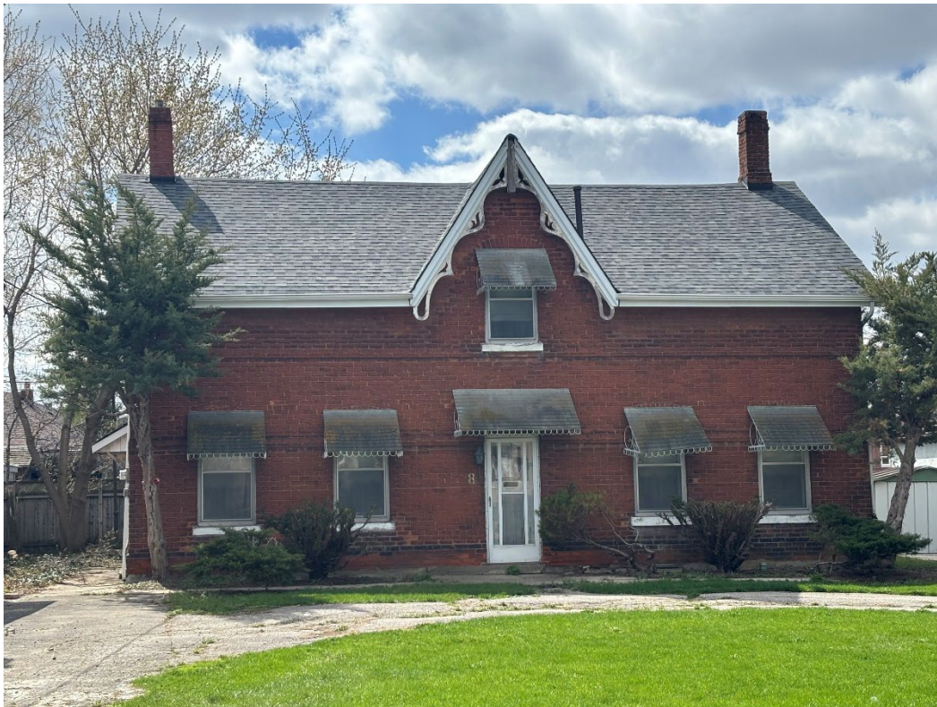
8 Arnold Avenue, view from the east (City of Toronto Heritage Planning, 2026)
