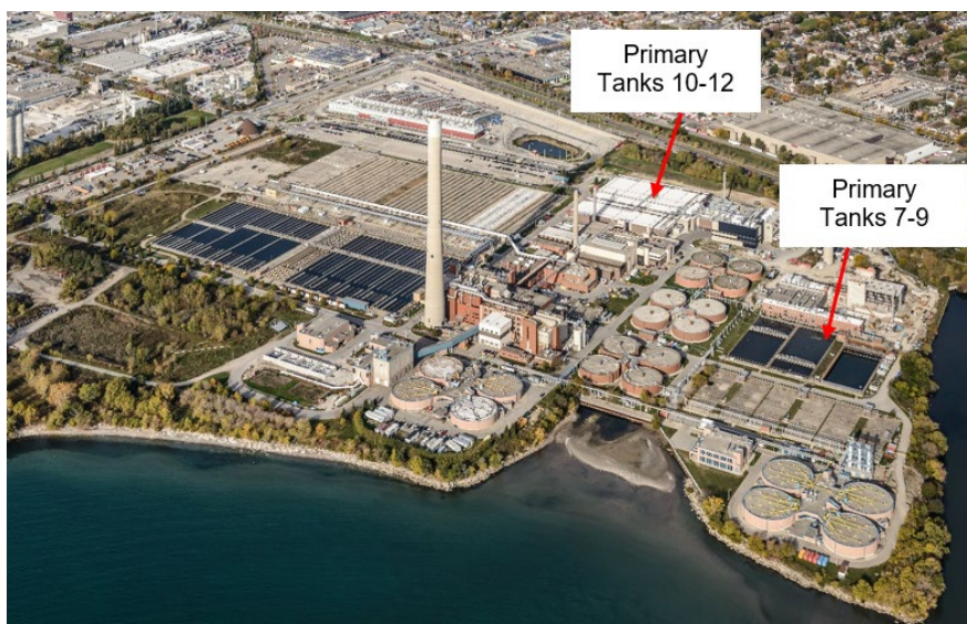
Figure 1 - Planned Tanks for Refurbishment at ABTP
