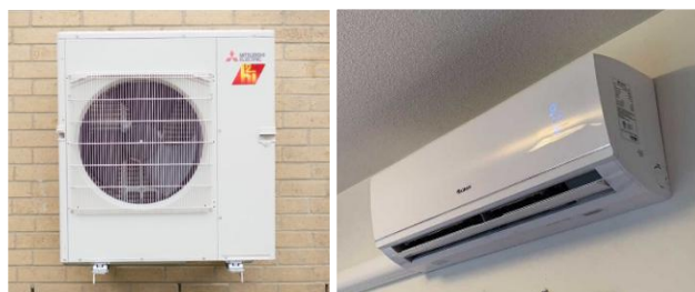
Figure 1: Left: Outdoor condensing unit portion of multi-/mini-split. Right: Wall mounted example of indoor portion of multi-/mini-split.
