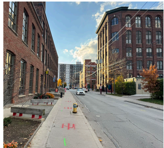
Fig. 1.20. Former Toronto Carpet Manufacturing Building (right) and subject property former S. F. Bowser and Company (left)
