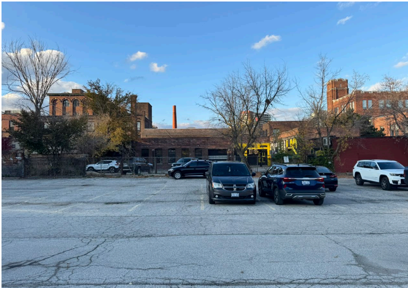
Fig. 1.15. View looking north towards the Site from an adjacent parking lot.
