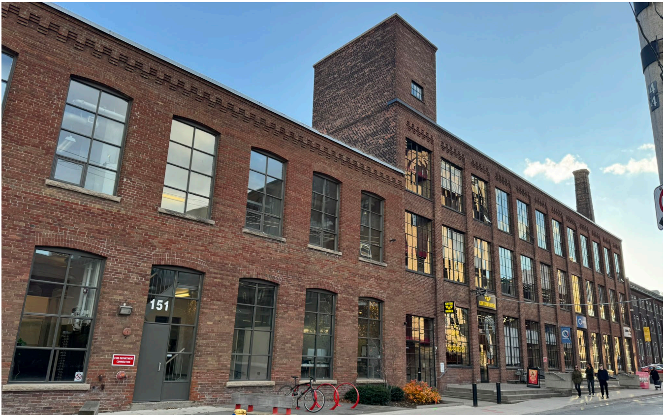
Fig. 1.9. Partial north elevation of 147 Liberty Street/ 68 Fraser Avenue (foreground) and 39 Mowat Avenue, former S. F. Bowser & Co addition, adjacent to it.
