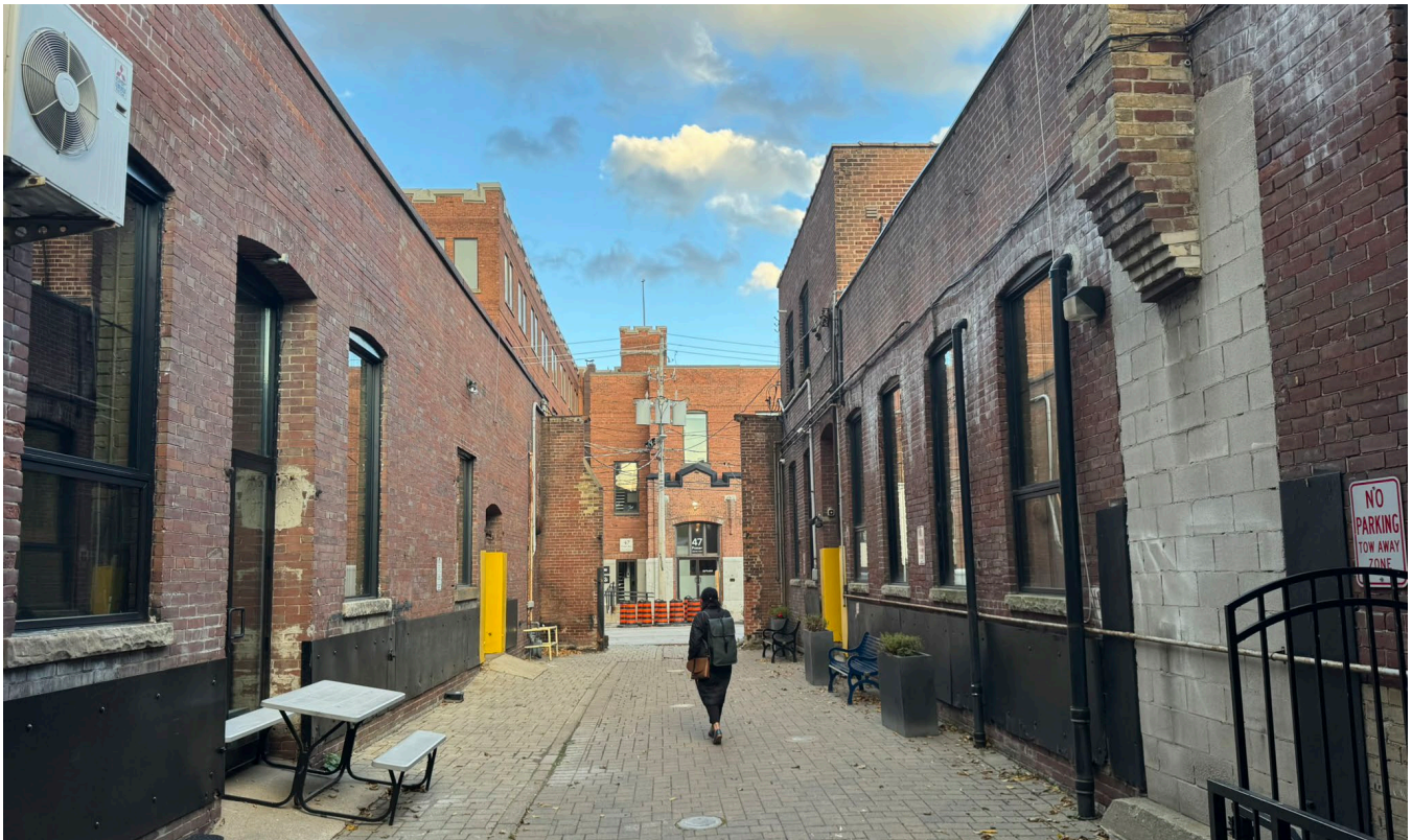
Fig. 1.12. Former Arlington Co courtyard, view looking east toward the Gillett Factory Complex.
