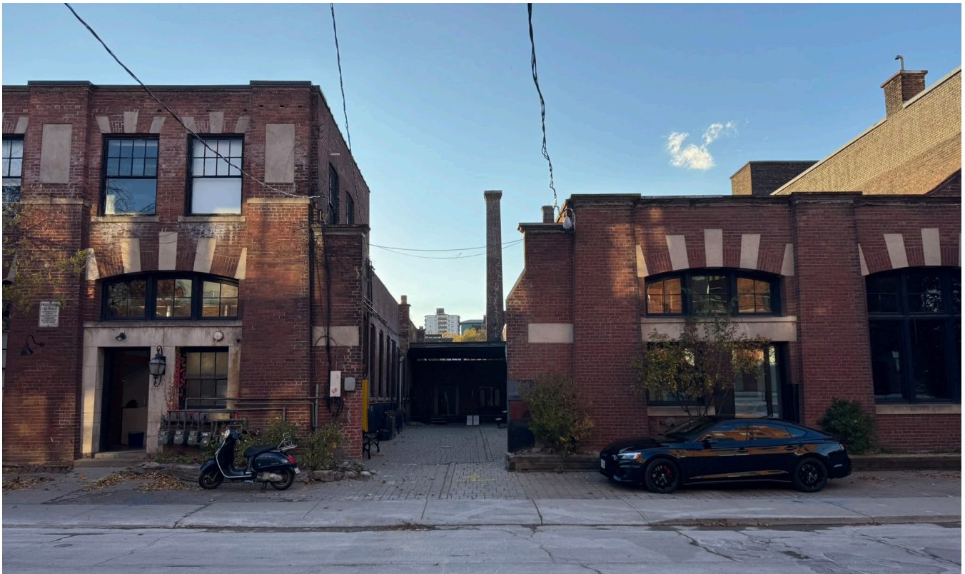
Fig. 1.10. 58-66 Fraser Avenue partial primary (east) elevation. South wing, courtyard and north wing of the former Arlington Co.
