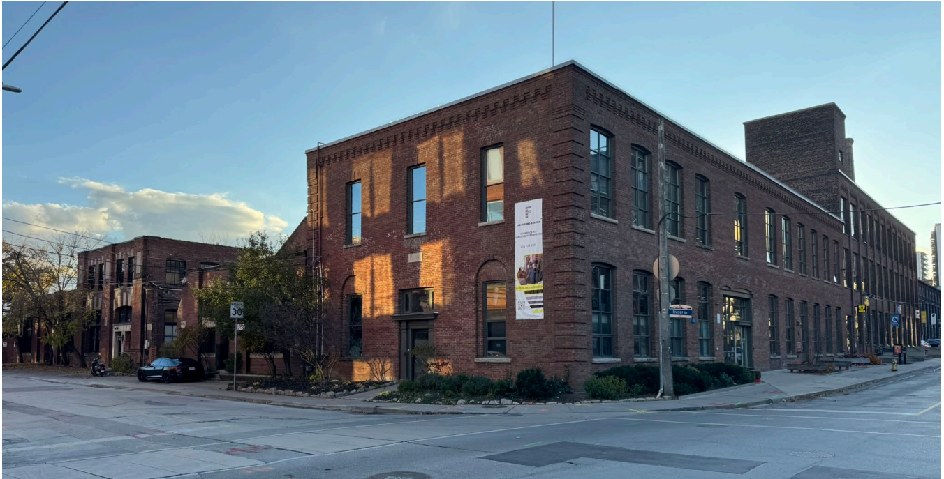
Fig. 1.6. East and north elevations of the former S. F. Bowser & Co factory at 147 Liberty Street/ 68 Fraser Avenue, looking towards the southwest Corner of Liberty Street and Fraser Avenue. 54-66 Fraser Avenue, the former Arlington Co, can also be seen in the background to the south.
