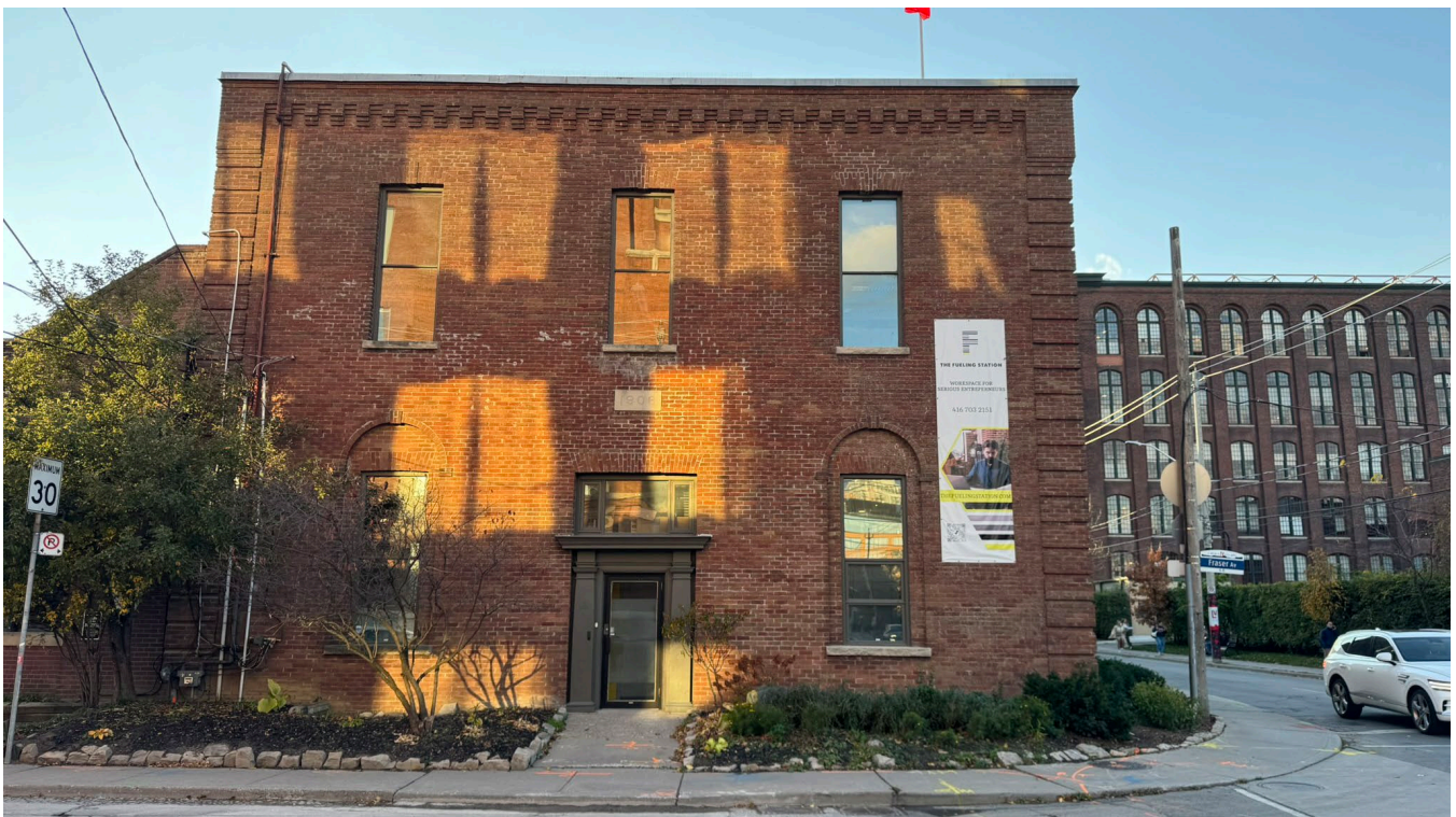
Fig. 1.7. 147 Liberty Street/ 68 Fraser Avenue east elevation which was historically main elevation.
