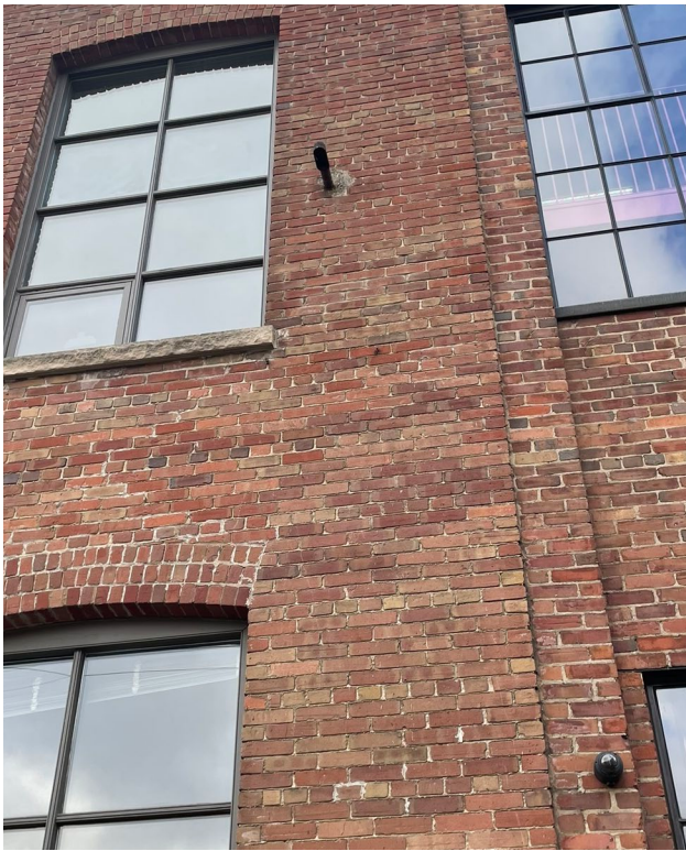
Fig. 5.1. North facade: example of general brick condition.
