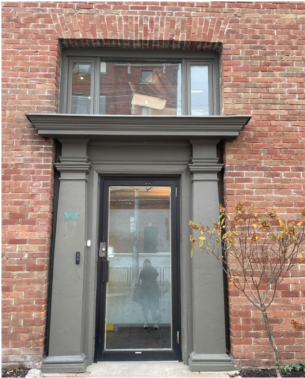
Fig. 5.13. East facade: brick condition at the main entrance showing minor mortar repairs.
