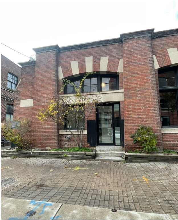
Fig. 5.15. East facade: southern bay of the original building, masonry in good condition.
