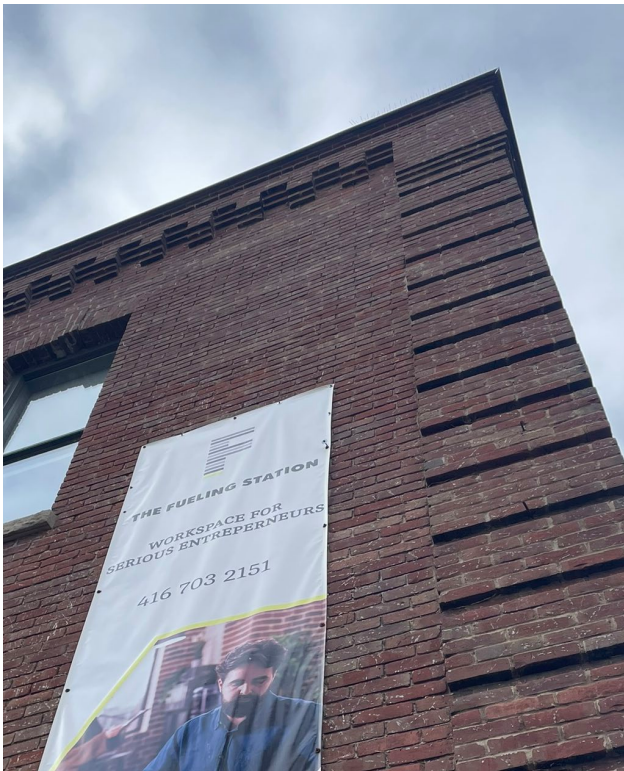
Fig. 5.7. North east corner: brick details in good condition.
