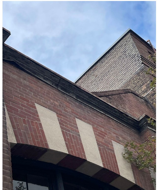
Fig. 5.20. East facade: brick and stone voussoirs at arched window openings in good condition.
