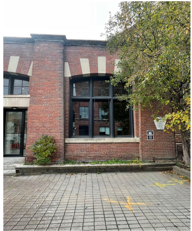
Fig. 5.16. East facade: northern bay of the original building, masonry in good condition.
