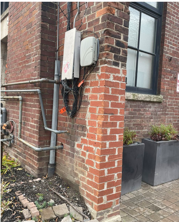
Fig. 5.21. East facade: entrance to the courtyard, example of brick repairs at former gate wall.
