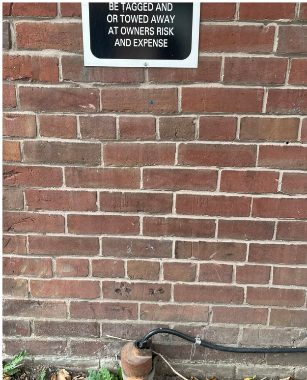
Fig. 5.17. East facade: example of general brick condition.
