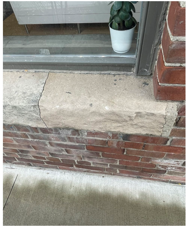
Fig. 5.6. North facade: example of repaired sill.
