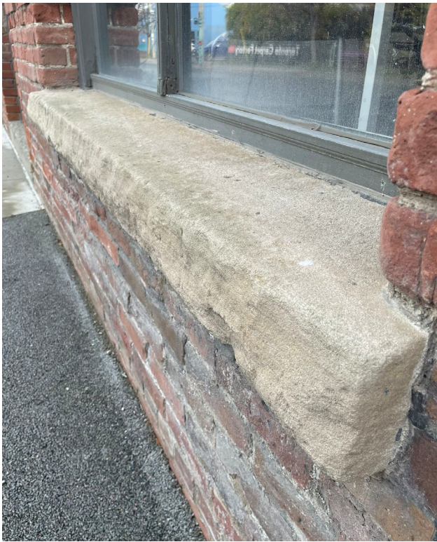
Fig. 5.5. North facade: example of stone sill condition.
