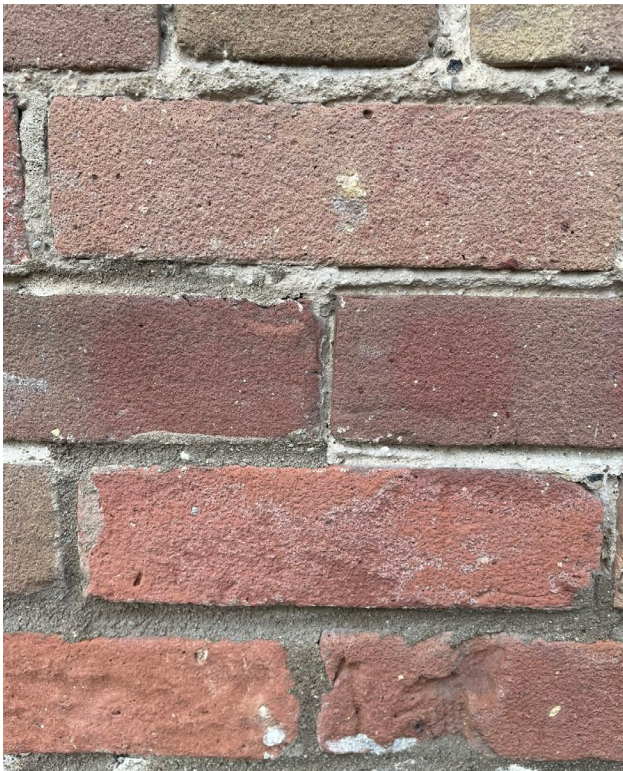
Fig. 5.3. Close up showing example of original and repair mortar.
