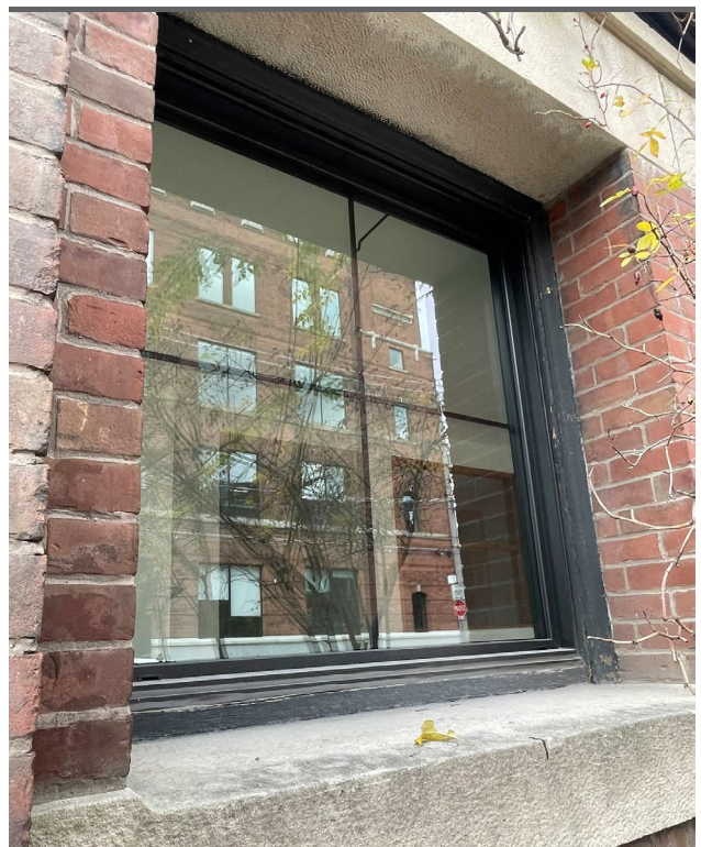
Fig. 5.22. East facade: example of replaced window sash. Limestone sills and lintels in good condition.
