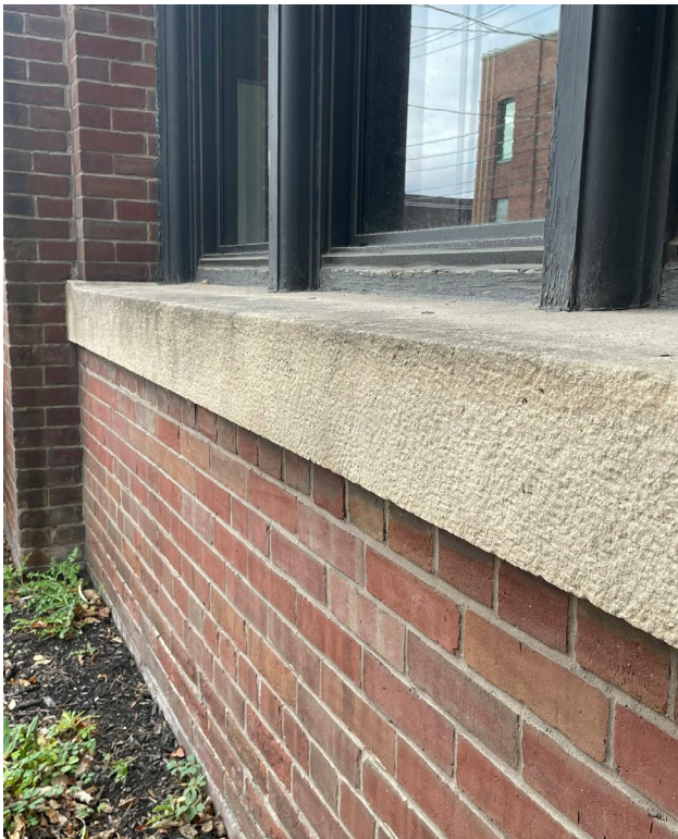
Fig. 5.19. East facade: sills in good condition with minor soiling.
