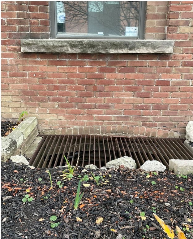
Fig. 5.14. East facade: example of general brick condition. Window wells are covered in metal screens.
