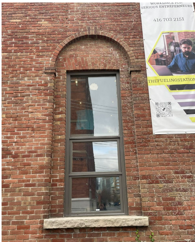
Fig. 5.11. East facade: brick in good condition at rounded-arch brick frames.
