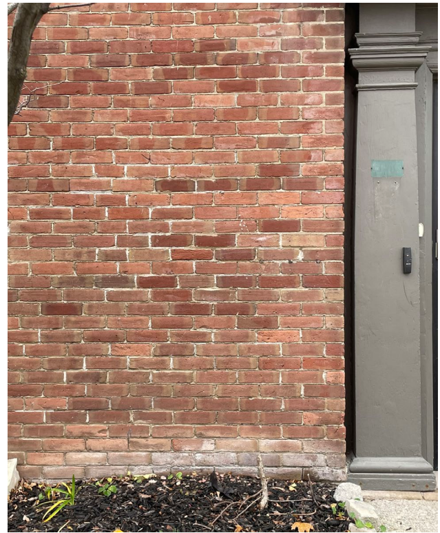
Fig. 5.10. East facade: example of brick condition.
