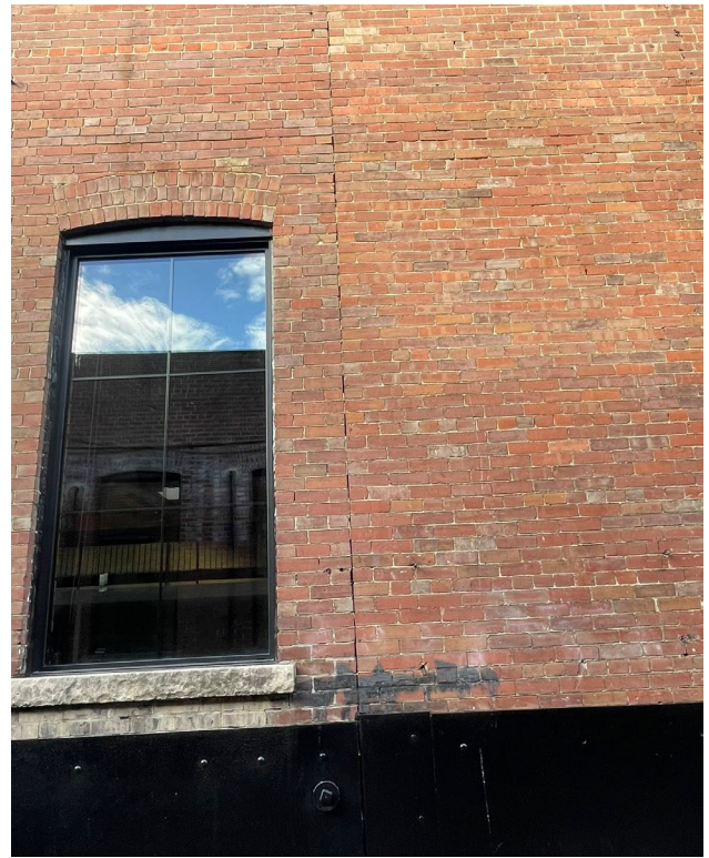
Fig. 5.32. Courtyard: line of one storey addition, and contemporaneity window replacements.
