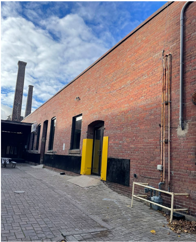
Fig. 5.31. Courtyard: masonry in fair condition.
