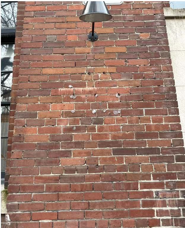
Fig. 5.25. East facade: example of mortar repairs at the southern bays.
