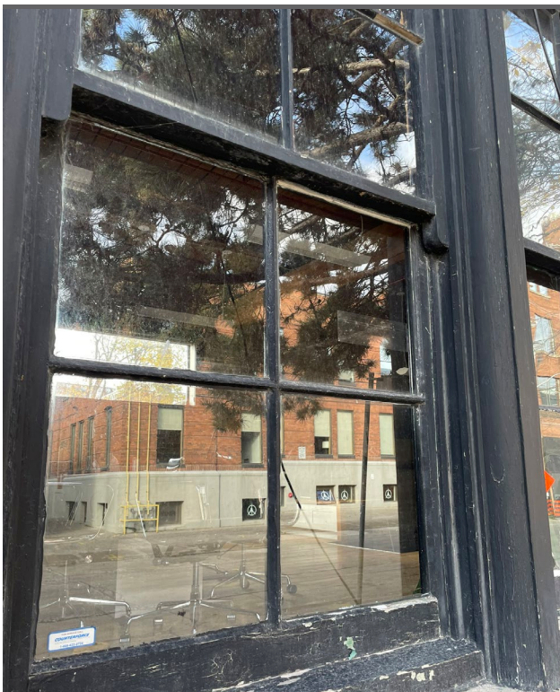
Fig. 5.29. Original wood windows in fair condition.
