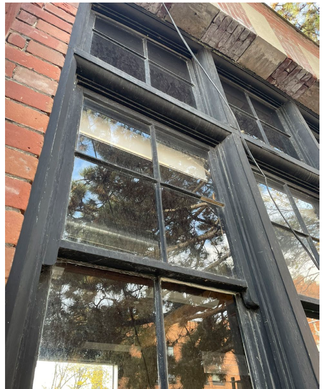
Fig. 5.30. Original wood windows in fair condition.
