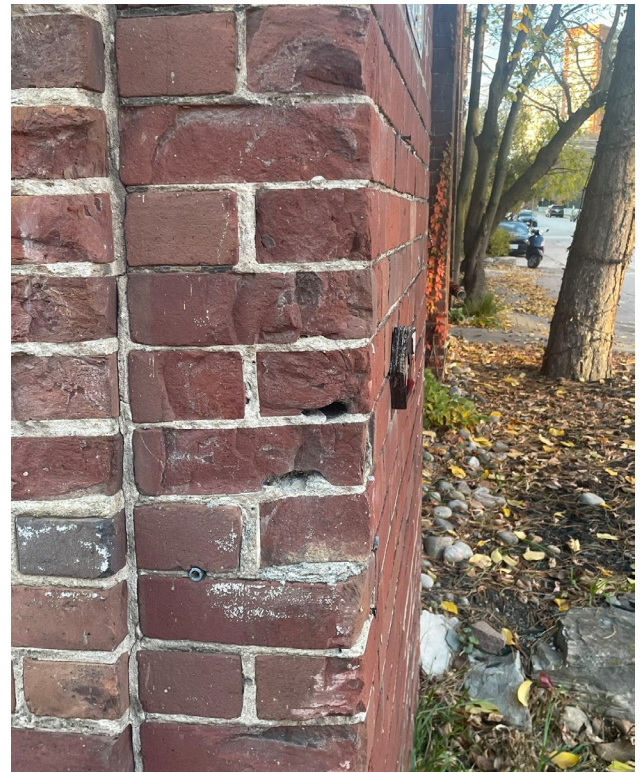
Fig. 5.51. Example of masonry condition at the corners.
