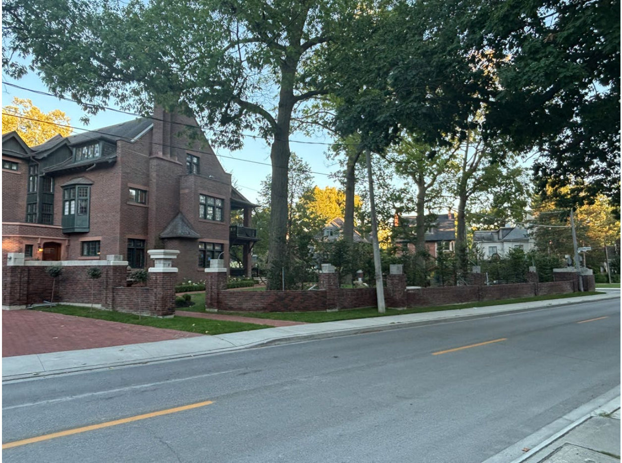
Figure 1: View of existing wall structure looking southeast toward 2 Whitney Avenue from Glen Road (City of Toronto, August 2025).
