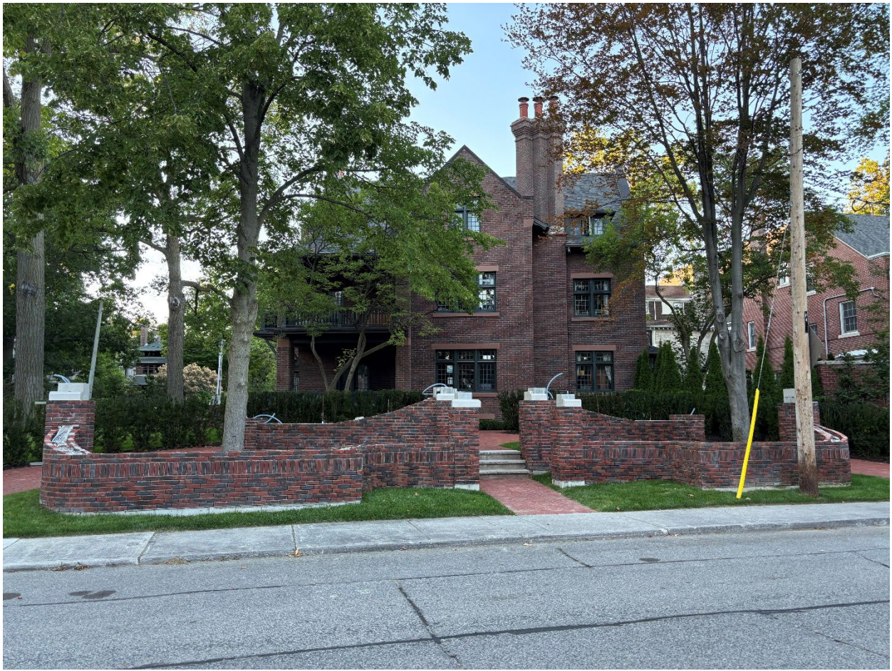
Figure 6: View of existing wall structure looking south towards 2 Whitney Avenue from Whitney Avenue (City of Toronto, August 2025).
