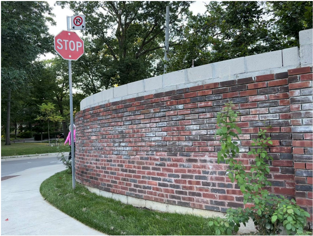
Figure 5: Detailed view of existing wall structure looking west towards Glen Road from corner of Glen Road and Whitney Avenue (City of Toronto, August 2025).
