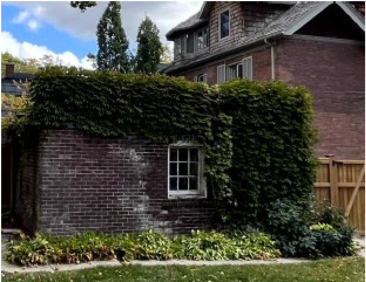
View of the west (side) elevation of the preexisting garage as seen from the rear yard at 6 Whitney Avenue (bsq Landscape Architects, 2026).
