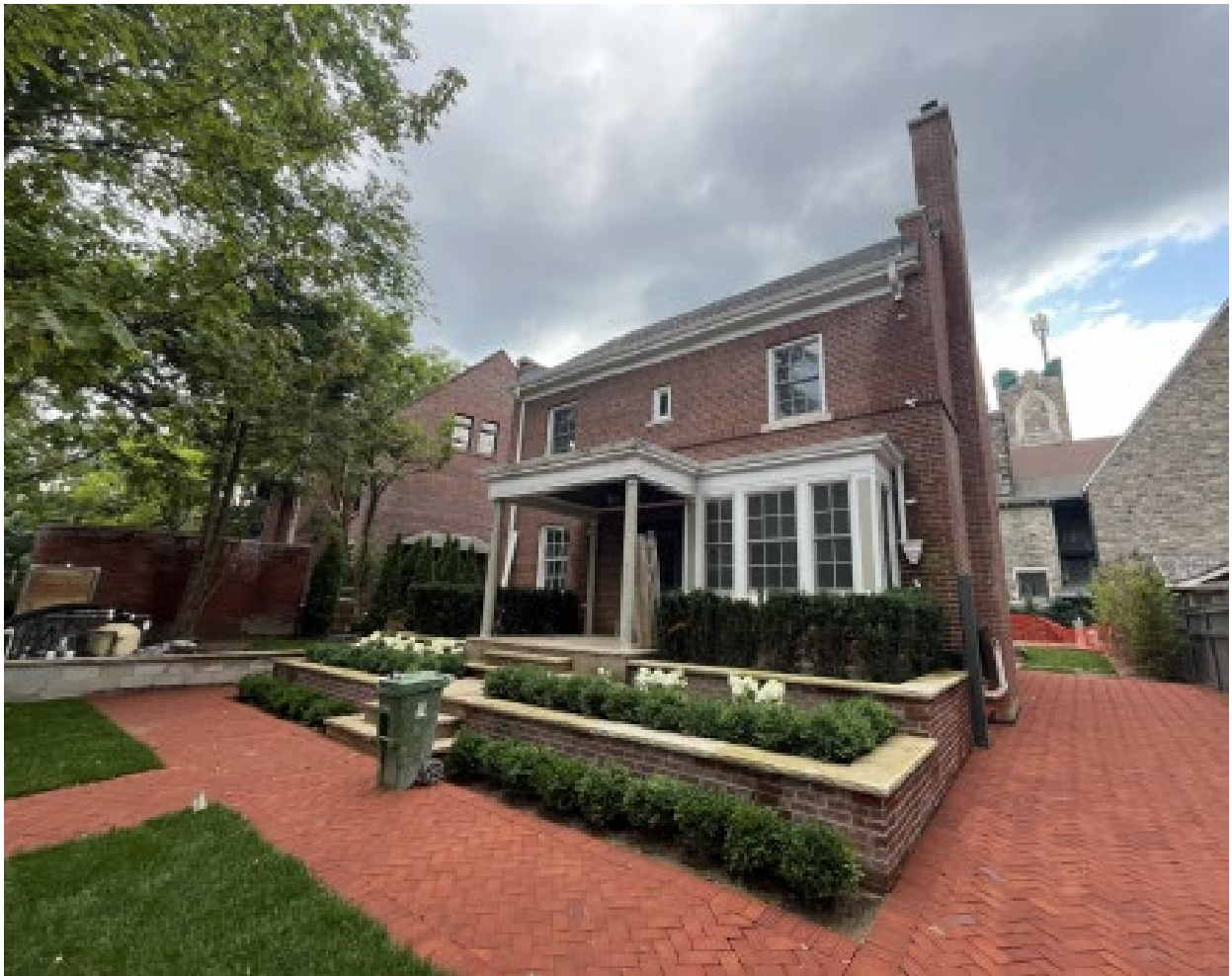
View of the principal elevation at 6 Whitney Avenue, showing existing context and preexisting garage demolished (bsq Landscape Architects, 2026).
