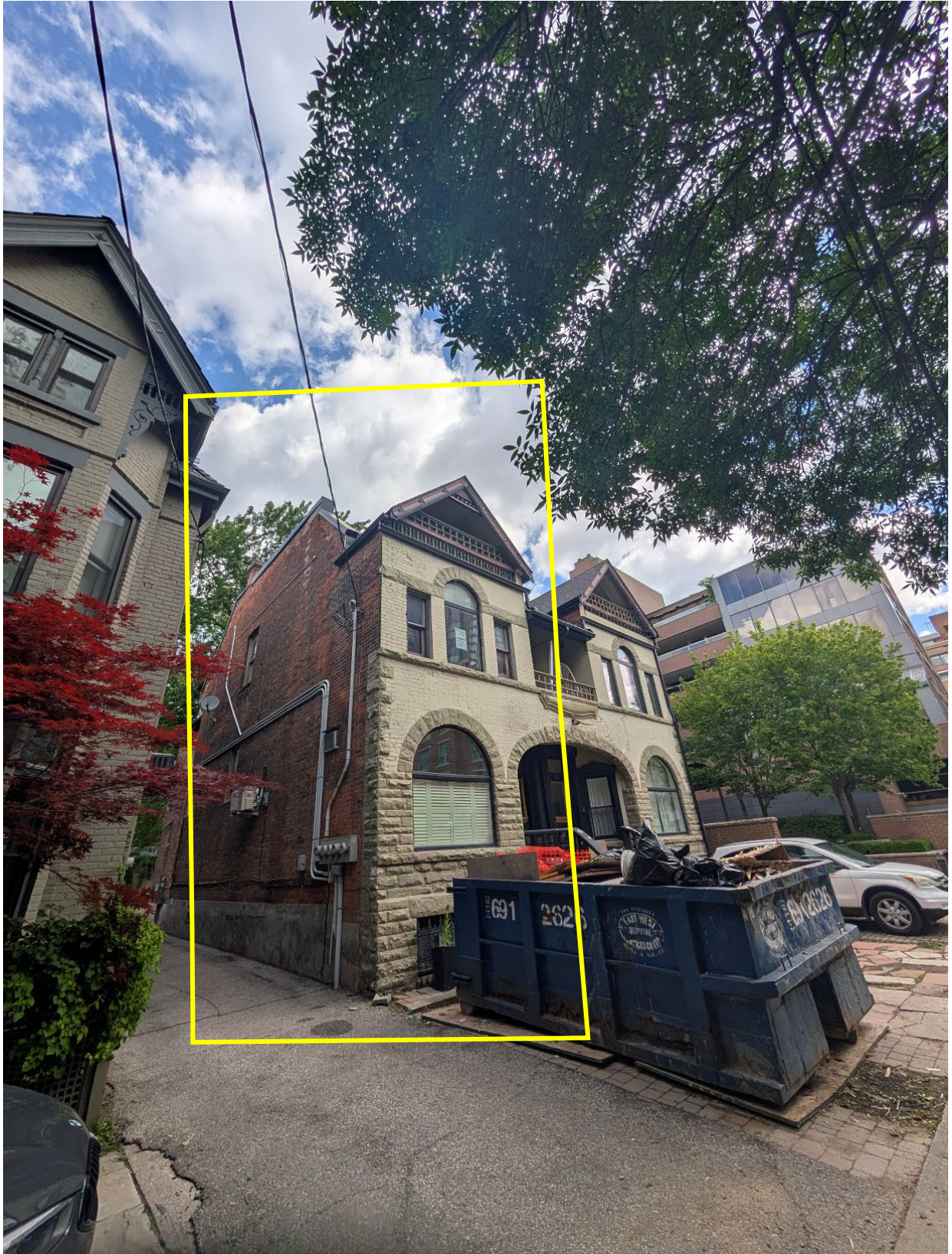
West elevation of 8 Lowther Avenue showing existing windows, doors and roof (Source: Heritage Planning, 2026)
