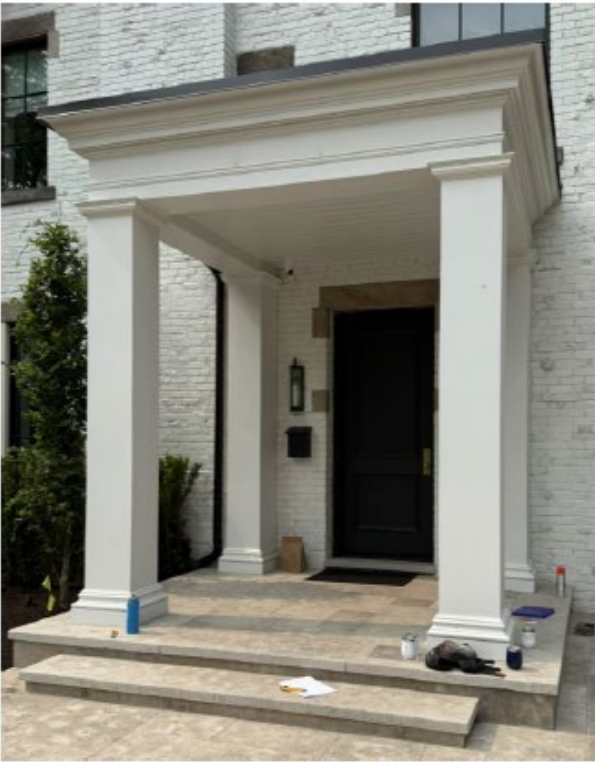
Figure 8 - New front porch at 87 Highland Avenue
