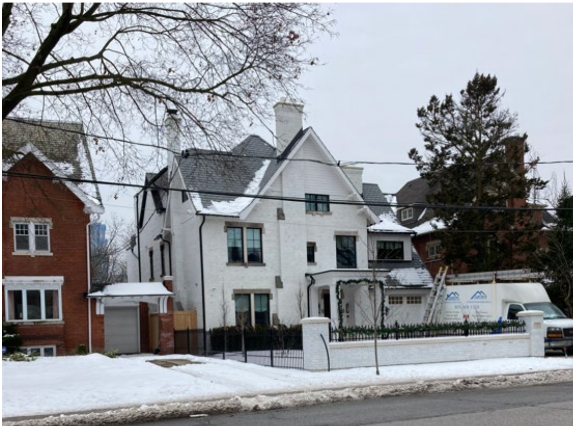
Photo of the northeast elevation of the existing building at 87 Highland Avenue after the unauthorized alterations (City of Toronto, 2025).
