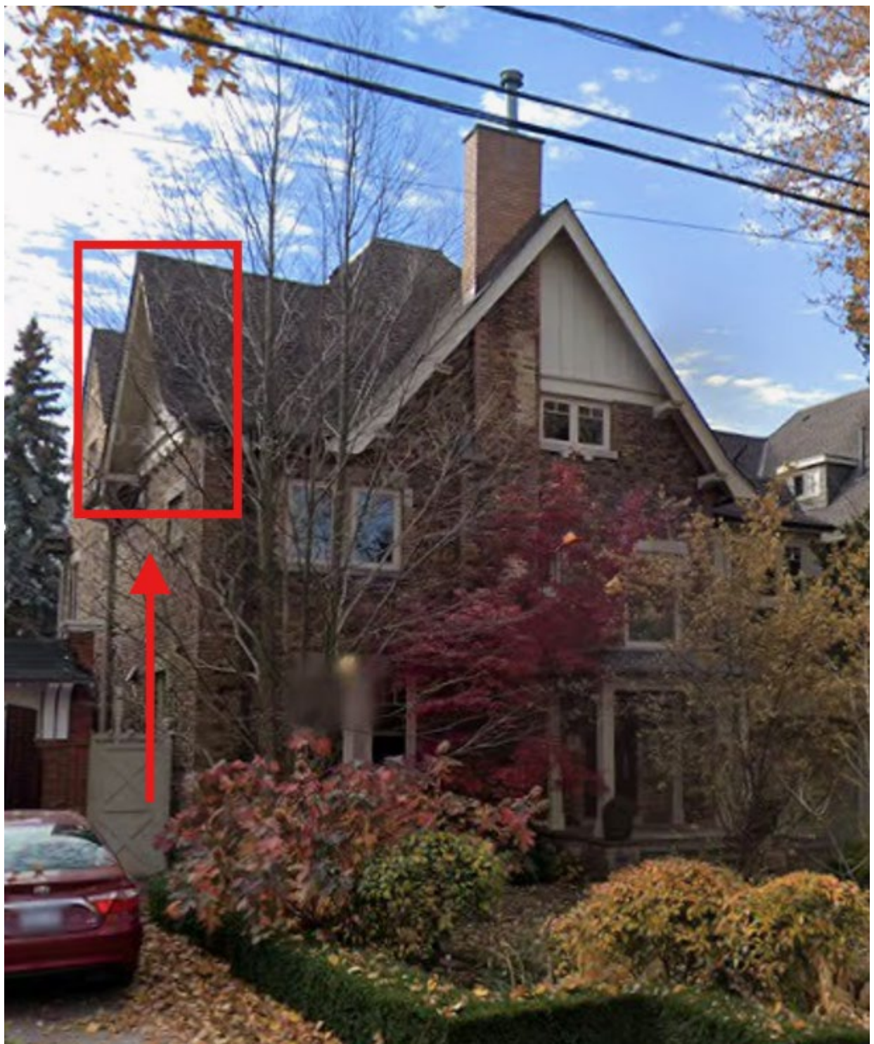
Photo of the northeast elevation of the existing building at 87 Highland Avenue showing architectural elements found on the east gable, prior to the unauthorized alterations (Google Maps, 2019)
