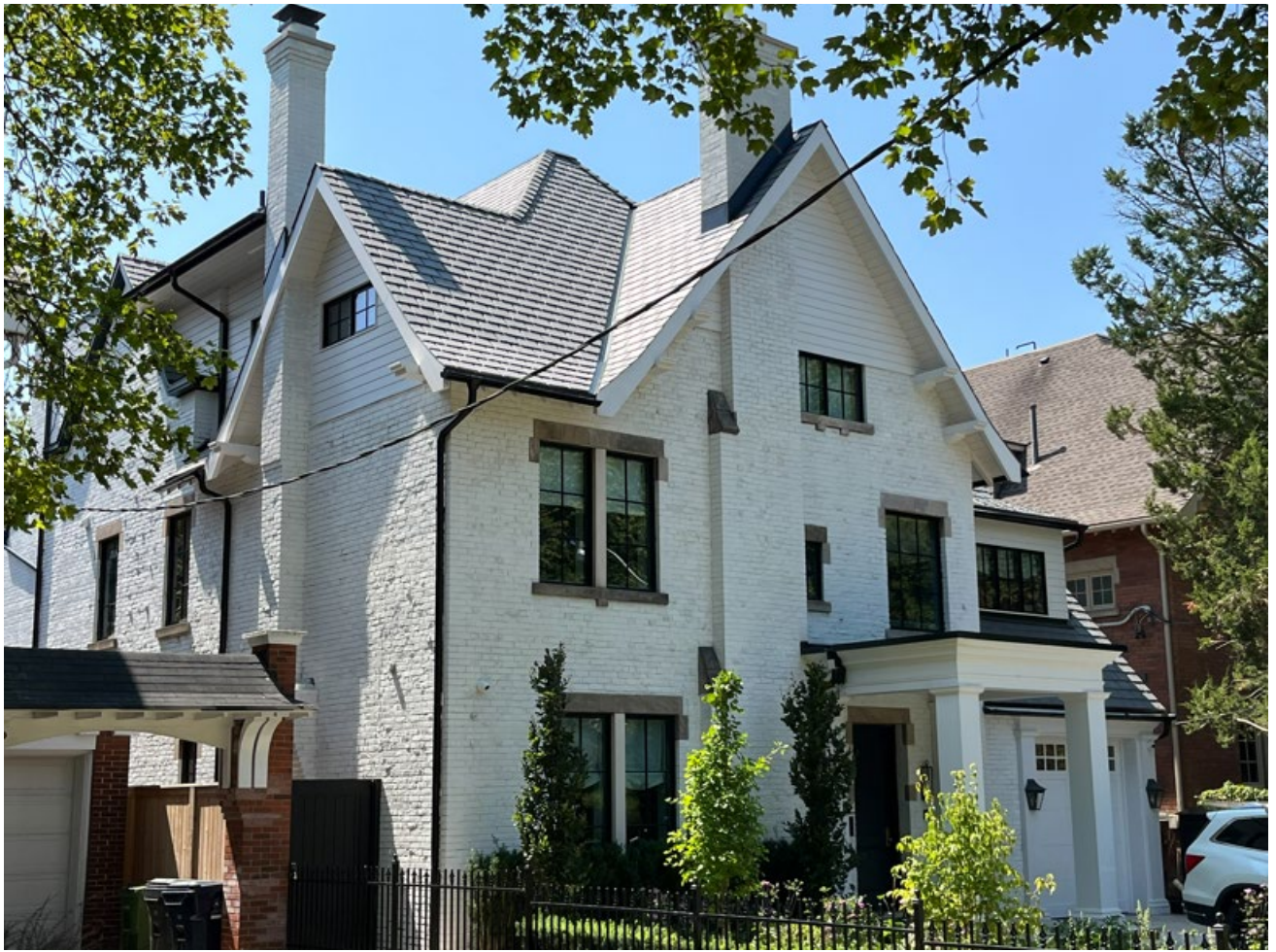
Detailed photo of the northeast elevation of the existing building at 87 Highland Avenue after the unauthorized alterations (City of Toronto, 2025).
