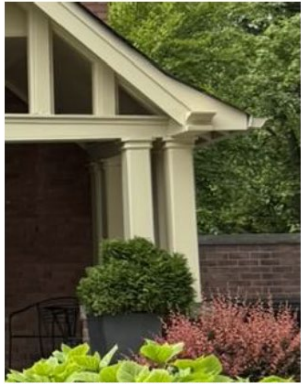
Figure 9 - Simple square porch columns at 85 Highland Avenue
