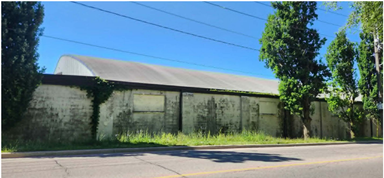
Figure 4: North façade, 2026 (City of Toronto Heritage Planning)
