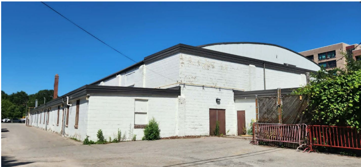
Figure 3: View of the rear (north) façade and one-storey south extension, 2026 (City of Toronto Heritage Planning)
