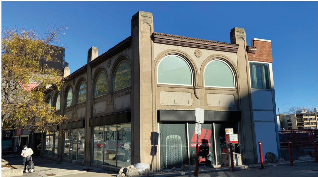
South Elevation of the heritage façade looking towards Yonge Street (ERA Architects, 2021)
