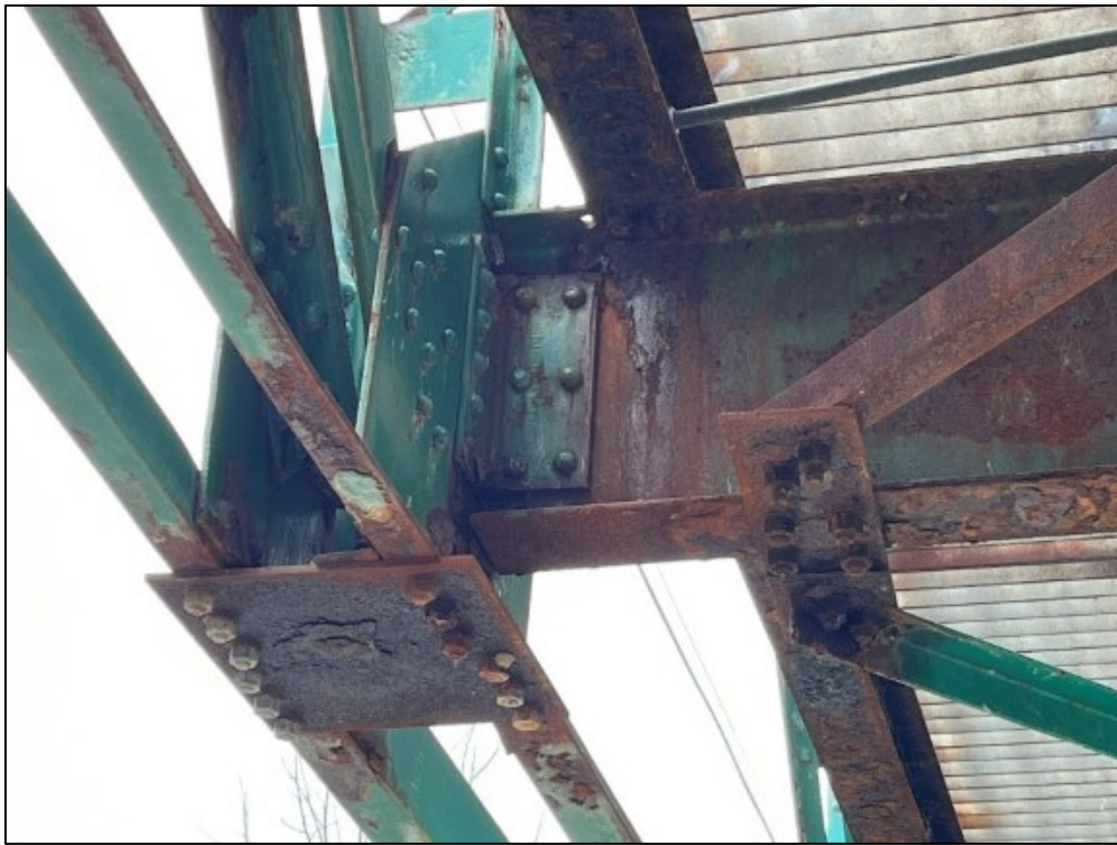
Detailed view of truss connections (ASI, 2025)
