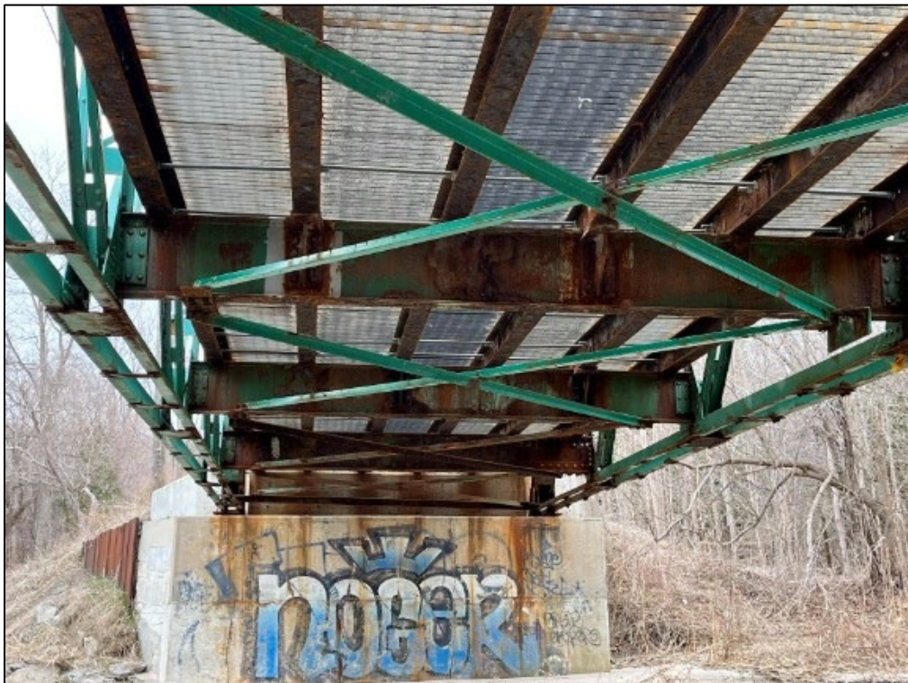
Interior soffit looking west, showing abutment, beams and stringers (ASI, 2025)
