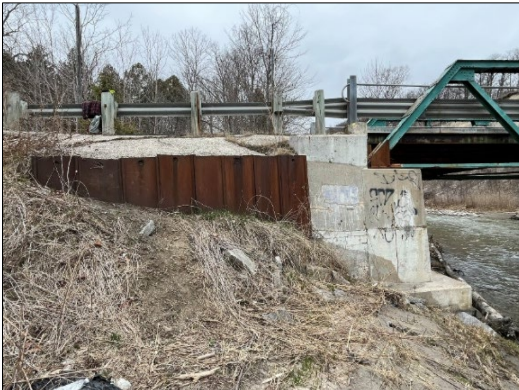
View of the southwest wingwall, looking north (ASI, 2025)
