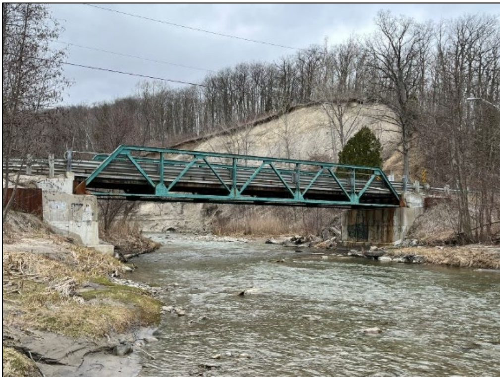
View of the south elevation of Stotts' Bridge, looking northeast (ASI, 2025)
