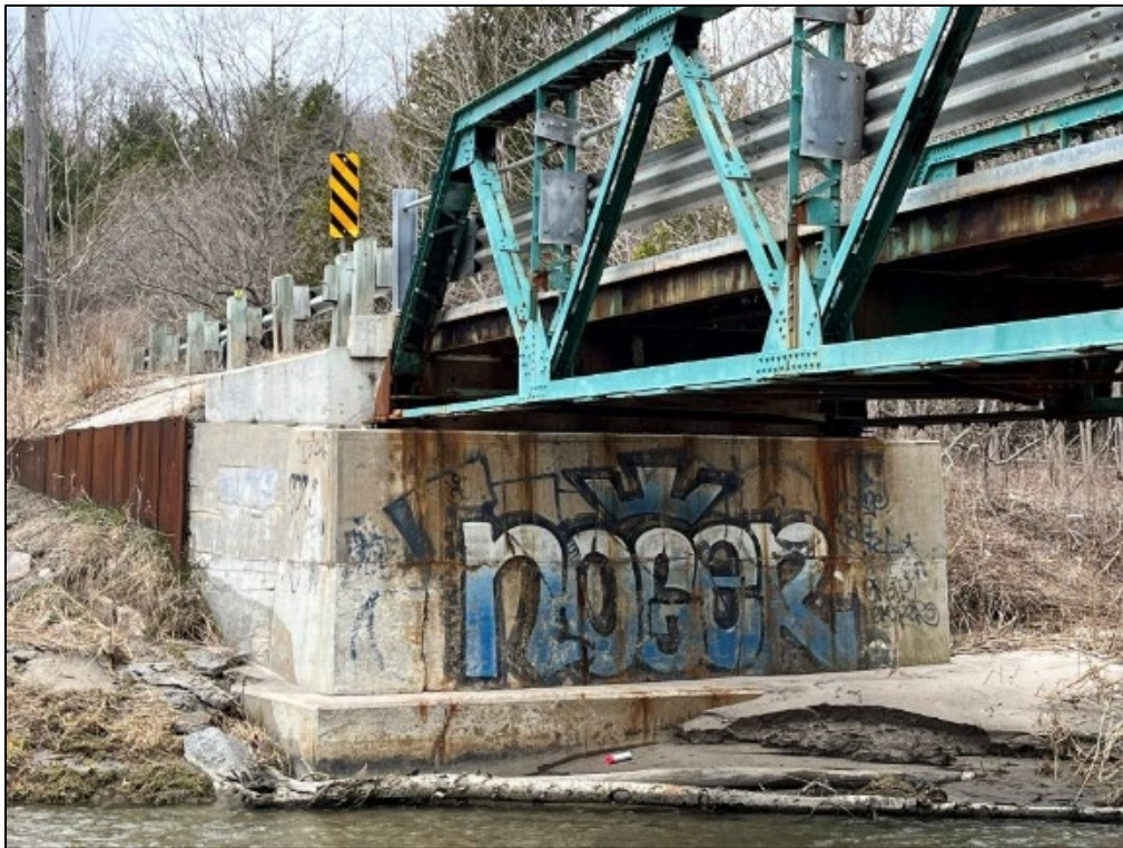
View of the west abutment wall, looking west (ASI, 2025)
